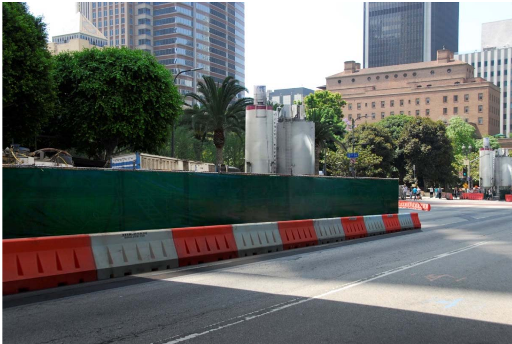
Figure 4.1-10: After View of Flower Street Facing Southeast North of 5th Street
