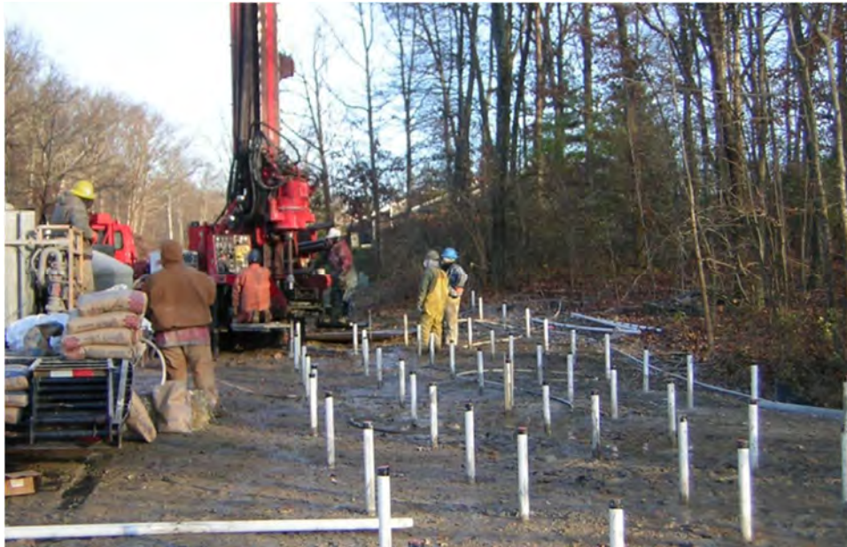
Figure 4-4: Permeation Grouting from Surface
