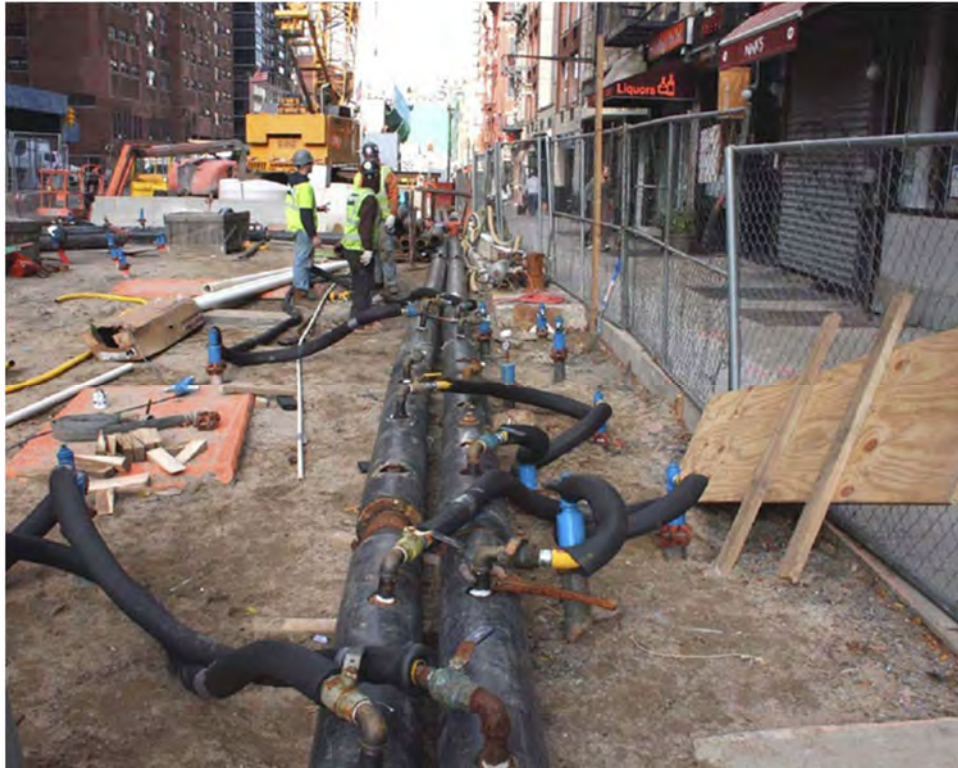
Figure 4-11: Ground Freezing Pipe Installation in New York City, Prior to Starting Freeze
