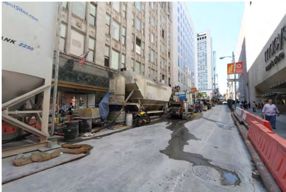
Figure 4-7: Staging for Jet Grouting Operation
