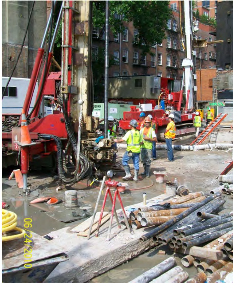
Figure 4-8: Surface Jet Grouting Operation
