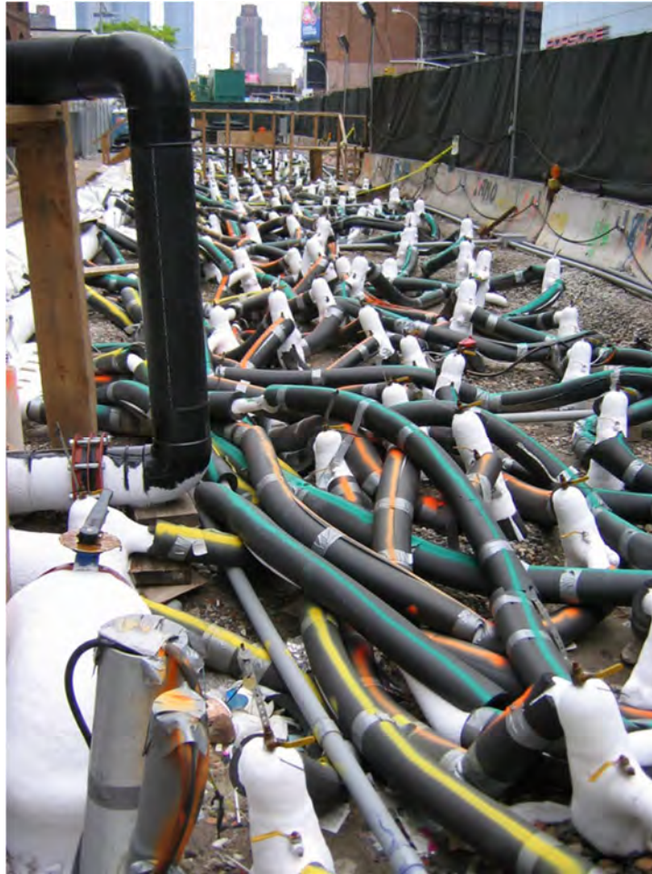
Figure 4-13: Freeze Pipe Array
