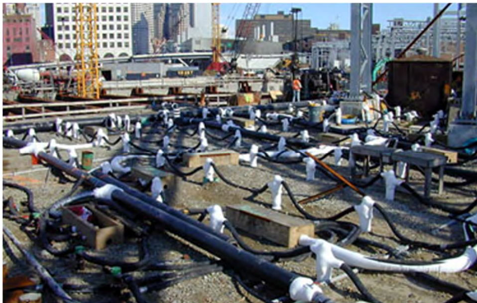
Figure 4-12: Ground Freezing Operation
