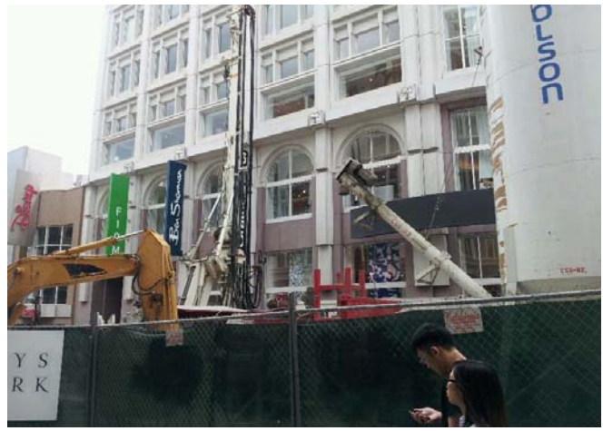
Figure 2.2-15: Grouting Equipment and Impacts (San Francisco, MUNI LRT Tunneling, 2013)
