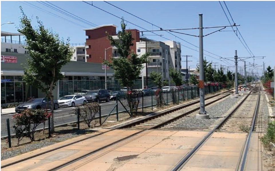
Figure 1-6. Example of Overhead Catenary System
