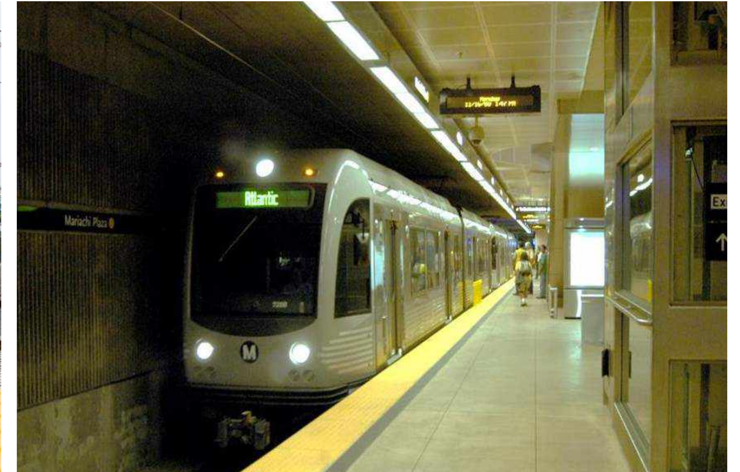
Underground: Gold Line – Mariachi Plaza
