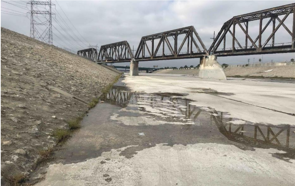
Photograph 3. Los Angeles River, facing south.
