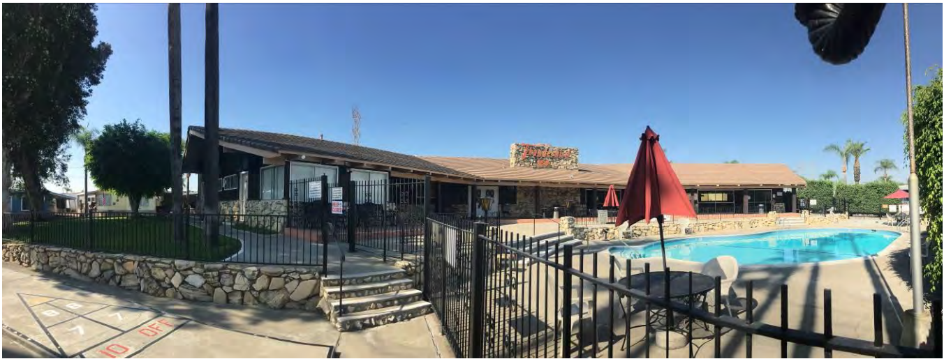
Clubhouse and swimming pool complex, west elevation. Camera facing northeast.
