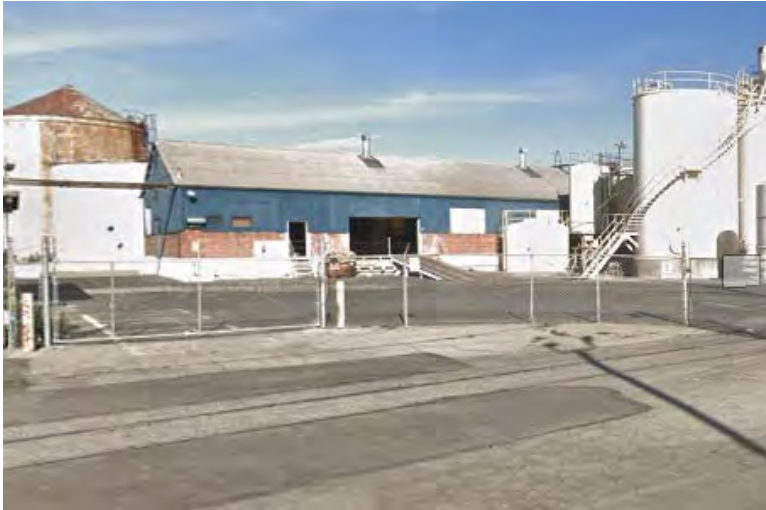
Figure 5. View of Building 4, east elevation, looking northwest
