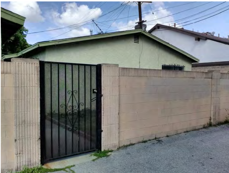
Photograph 3. Obstructed view of rear residence, south and east elevations.
