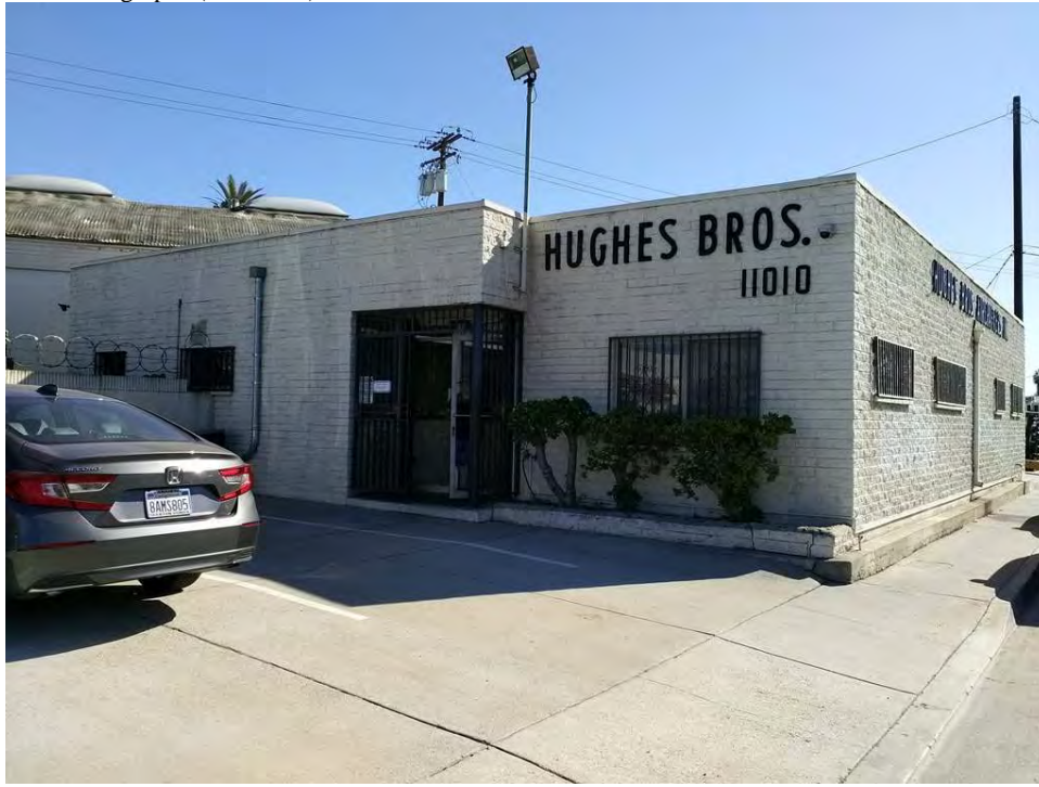
Photograph 2. Office building, north and west elevations. Camera facing southeast.
