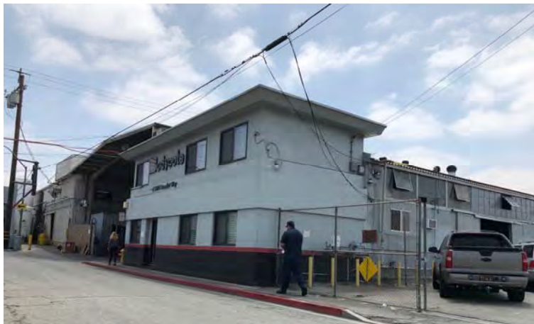
3370 Benedict Way, north and west elevation, view east
