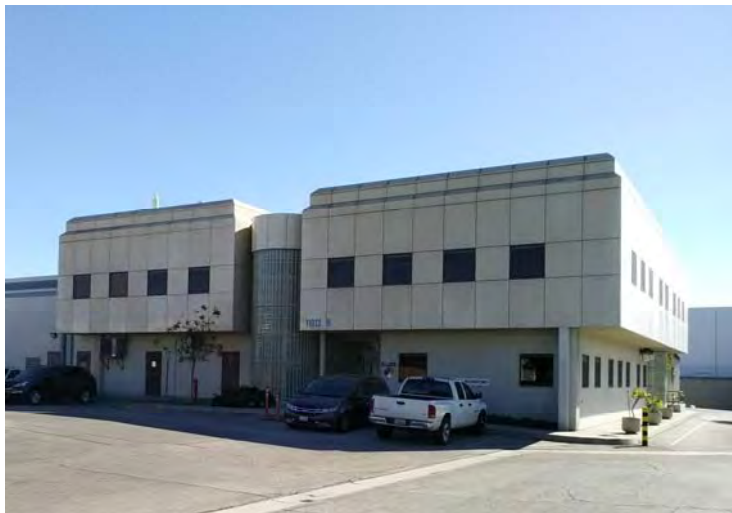
Central building (unknown use), north and west elevations, view to southeast
