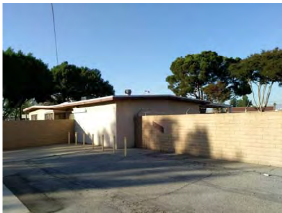
Building at southwest corner of the property, view to the northwest.
