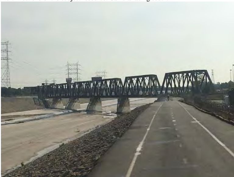
Overview of subject resource. Camera facing north.
