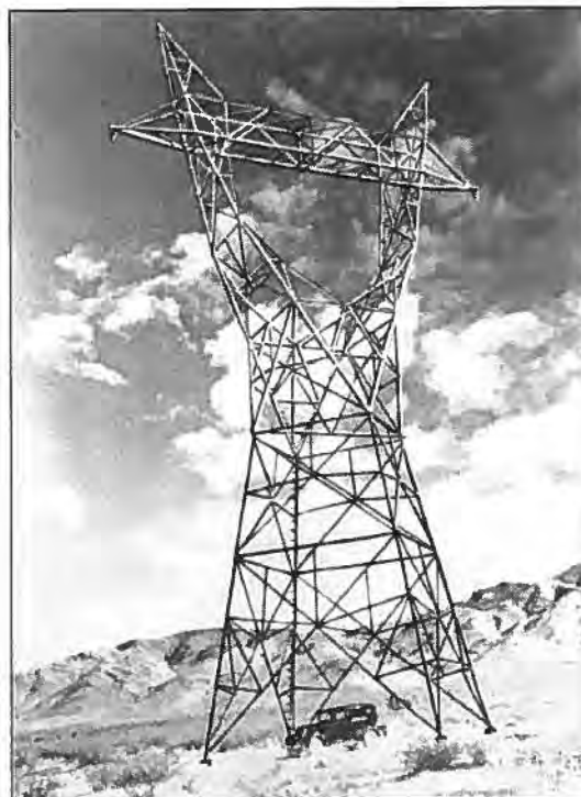
Figure 2: Example of the standard single circuit towers, ca. 1935. From the Historical Photo Collection of the Department of Water and Power, City of Los Angeles.
