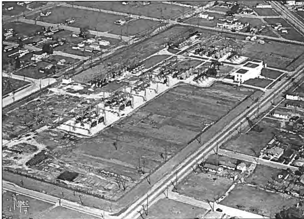
Figure 3: Aerial photograph of the Century Receiving Station showing the control house on the upper right, the oil house center left and the yard, ca. 1935. From the Historical Photo Collection of the Department of Water and Power, City of Los Angeles.
