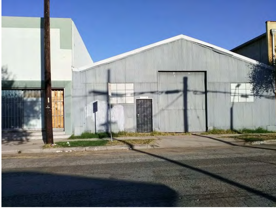
Photograph 2. South building (11710 Center Street), west elevation. Camera facing east.
