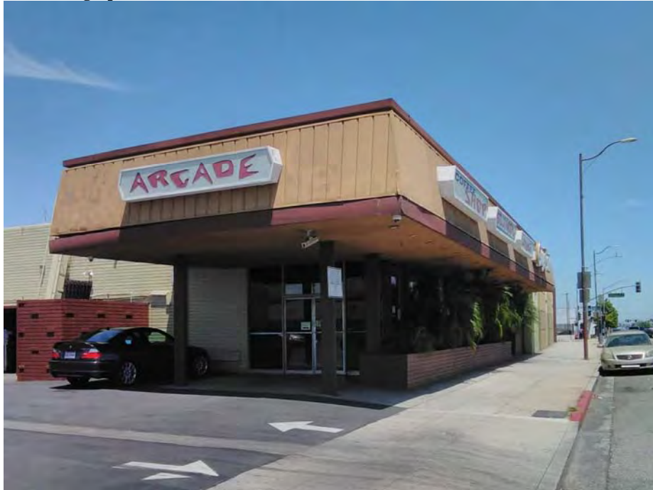
Photograph 2. South and west elevations. Camera facing northeast.
