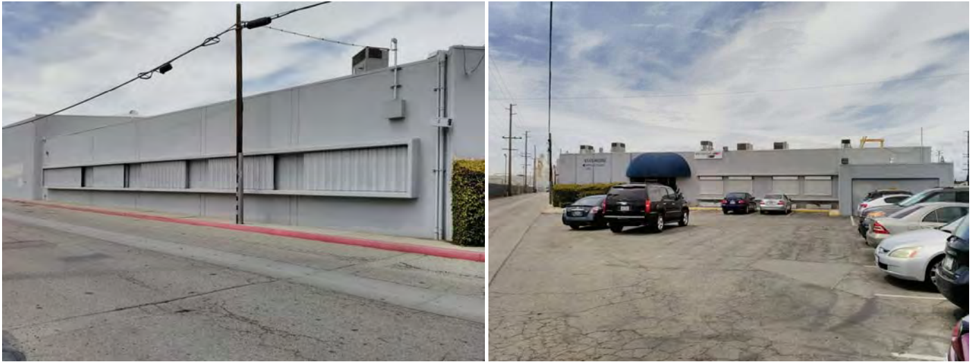
Figure 6. View of Building 6
