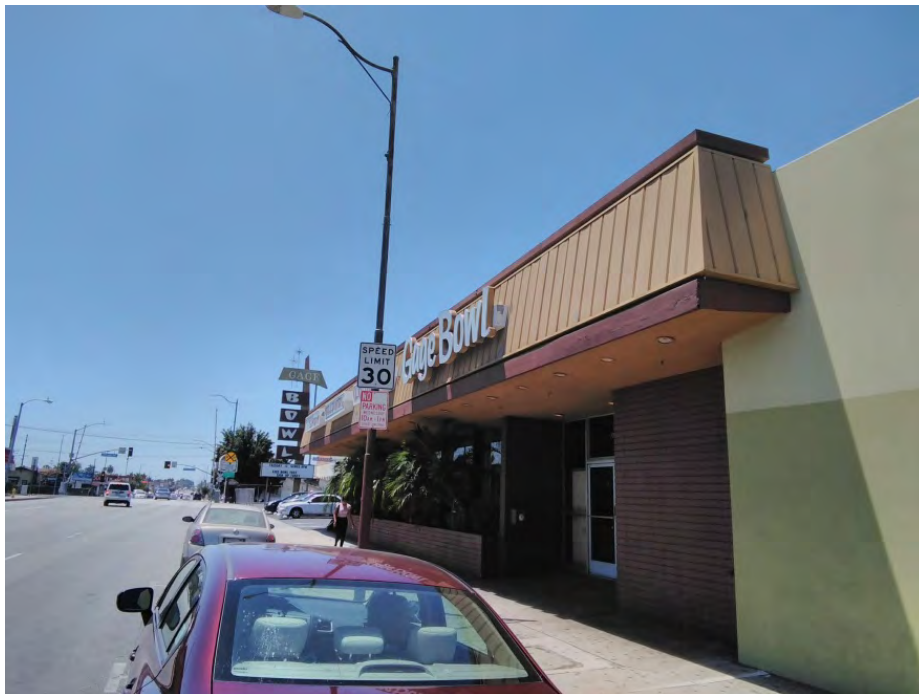
Photograph 3. South elevation with sign in the background. Camera facing northeast.
