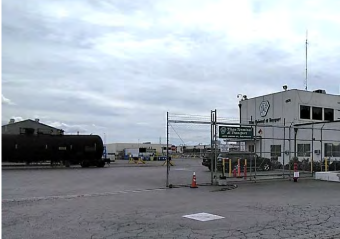
Figure 2. View of storage facility (left) and administrative building (right)
