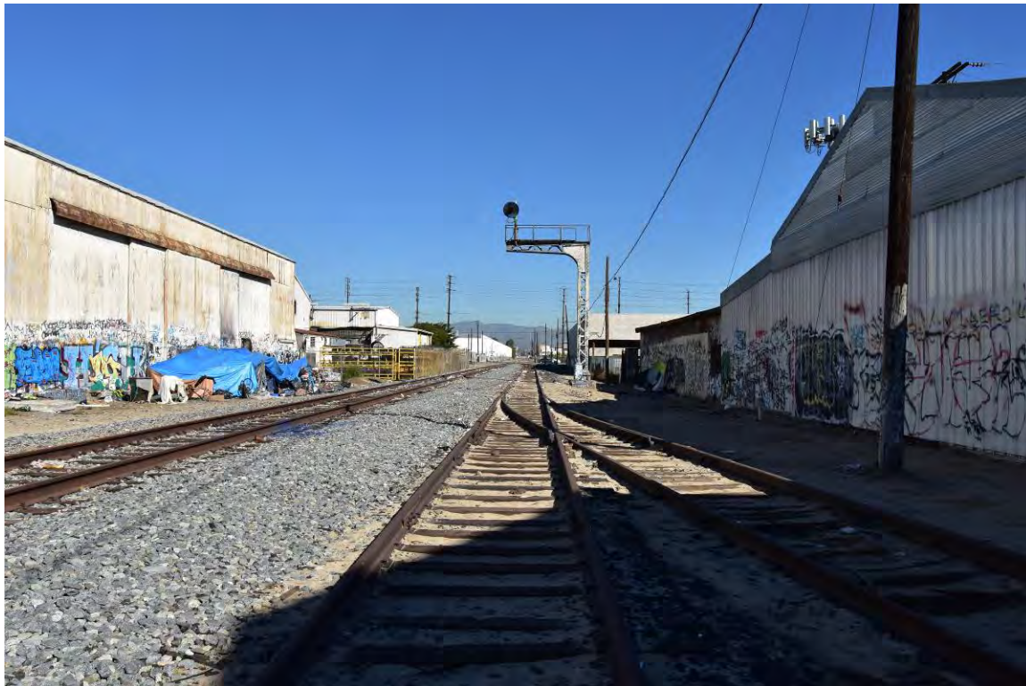
LATR tracks with elevated signal north of LATR and Pacific Electric Whittier Line junction. Camera facing south.
