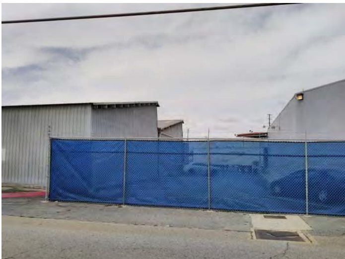
Figure 5. View of Building 5 (left) and 6 (right)
