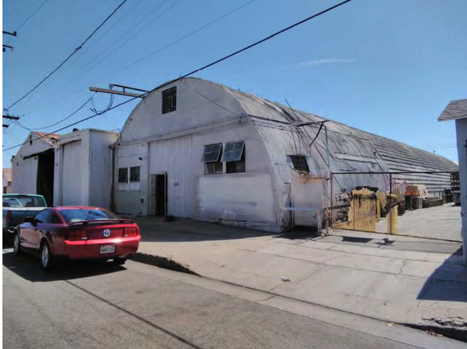
Photograph 3. Quonset hut (center) and Butler building (left), north and east elevations. Camera facing southwest.
