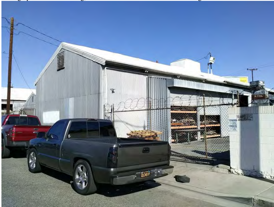
Photograph 3. Representative warehouse, south and west elevations. Camera facing northeast.
