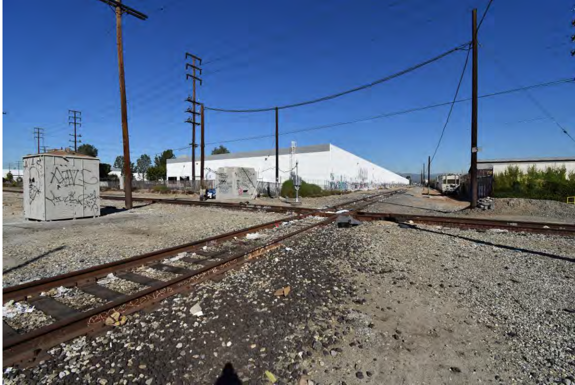
Junction of LATR and Pacific Electric Whittier Line tracks. Camera facing northwest.
