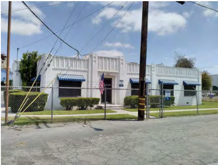
Figure 6. View of Building 2, south elevation, looking northeast
