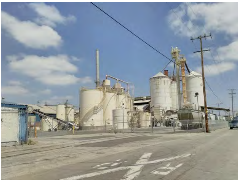
Figure 4. View of parts of Buildings 4, 5 and tanks, looking northwest
