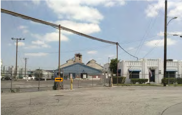
Figure 3. View of Building 1 (left) and Building 2 (right), looking north
