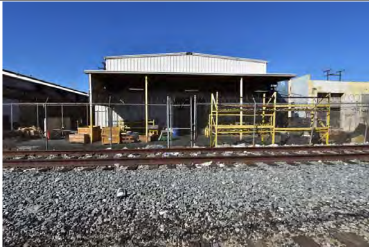
6304 Bissell Place, east elevation, view west.
