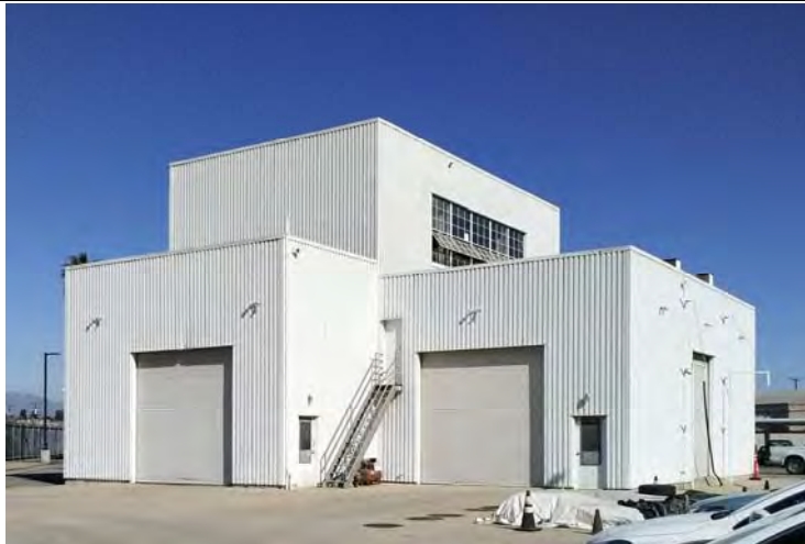
Northernmost building (unknown use), west and south elevations, view to northeast
