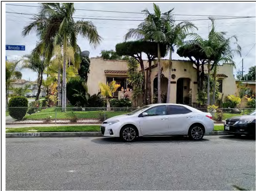
P5b. Description of Photo: North façade; camera facing south.
