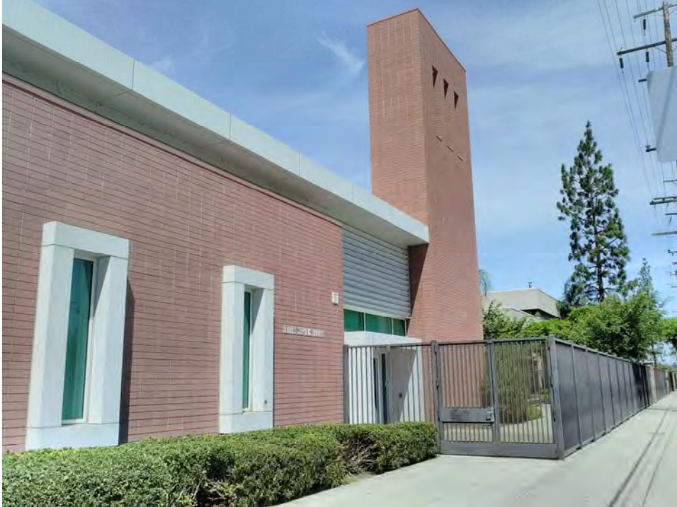
Photograph 4. Library, east elevation. Camera facing northeast.
