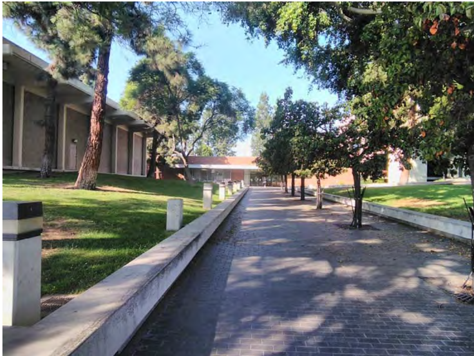
Health Building façade and east elevation of the library; north-facing
