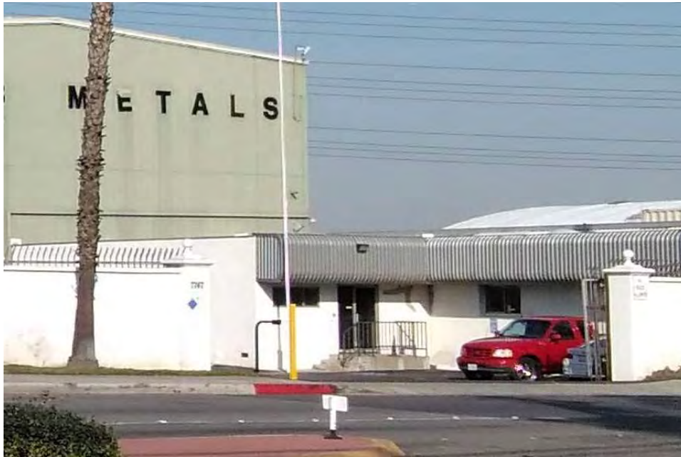
Easternmost office building, south and west elevations, view northeast.
