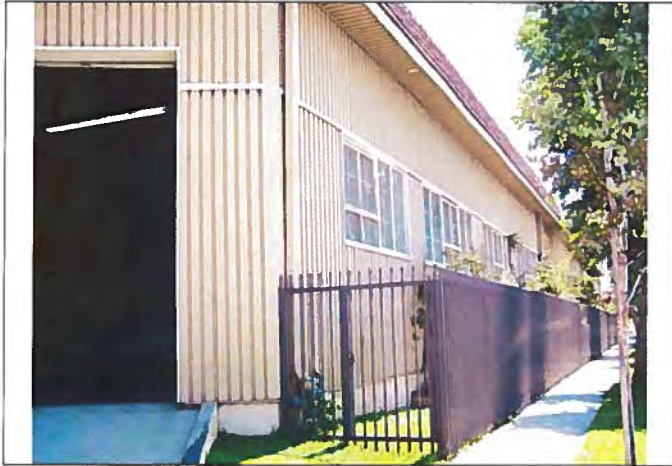
View looking northeast at the south elevation of the 1946 addition.
