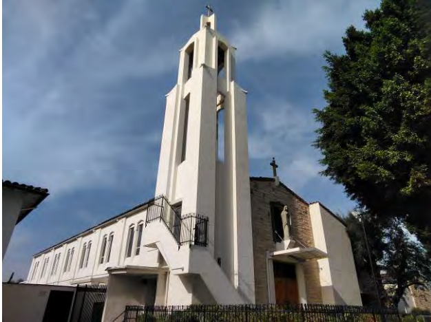
Church, eastern façade, view northwest.
