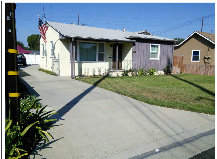
P5b. Description of Photo: South elevation of building, camera facing northeast
