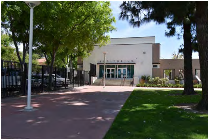
Paramount Park High School West Auditorium Building (Building #6), West (primary) Elevation; East-facing
