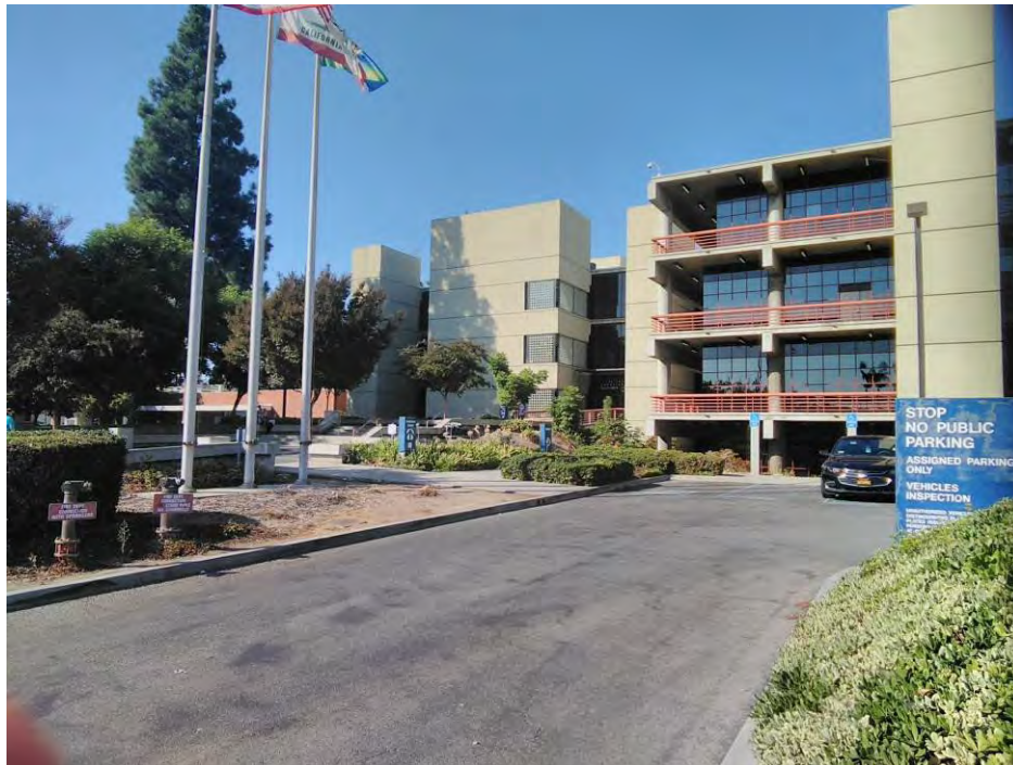
Los Angeles Superior Court-Bellflower Courthouse, south elevation; north-facing
