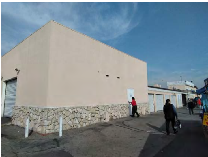
Southwest corner of projector/concessions building, view to the north
