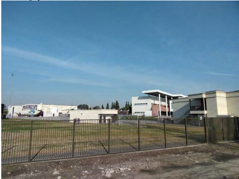
Photograph 2. Overview of south end of PHS West Campus: (left to right): Gymnasium, restroom, Medical Health and Science Building, classroom building. Camera facing northeast.
