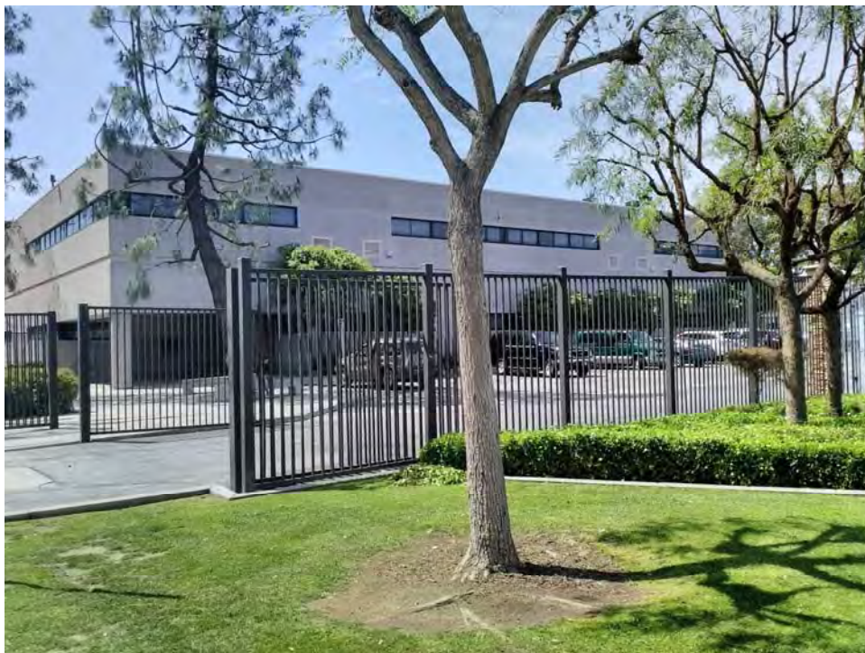
Photograph 3. Two-story classroom building, north and east elevations. Camera facing southwest.
