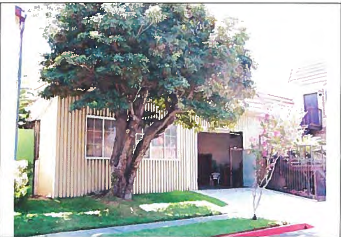
View looking southeast at the west elevation of the building
