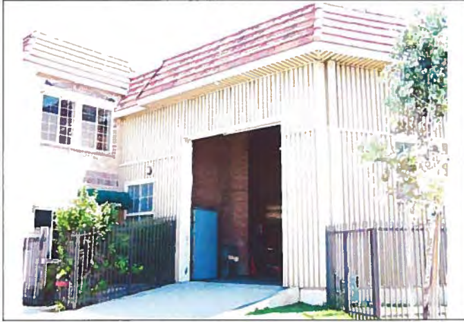
View looking northeast at the entrance to the 1946 addition.
