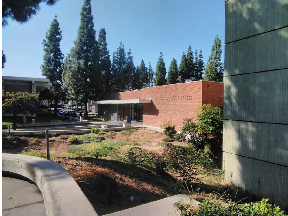
Health building and library, view to the southwest
