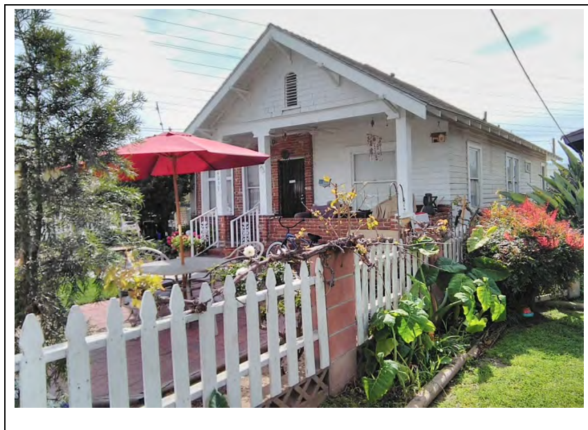
P5b. Description of Photo: Eastern façade and north elevation, view southwest, January 2018.
