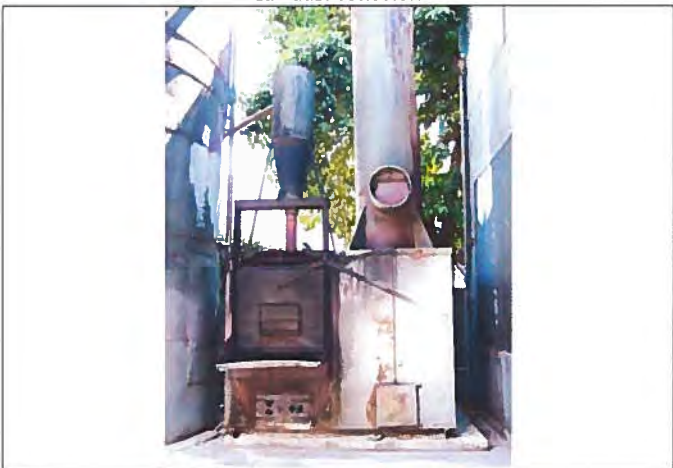
View looking east at the base of the circa 1970s incinerator.
