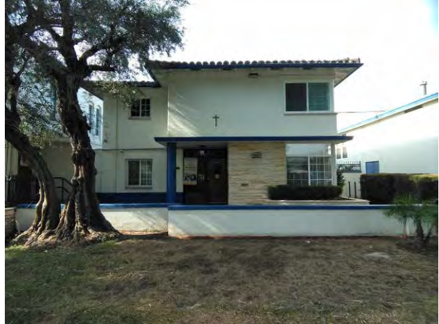
Rectory building, eastern façade, view west.
