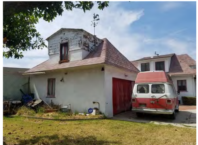
Garage, south and east elevations (Source: Redfin real estate listing, 2018).
