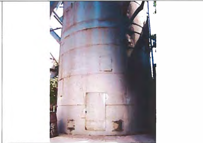
View looking east at the base of the 1957 sawdust collector.
