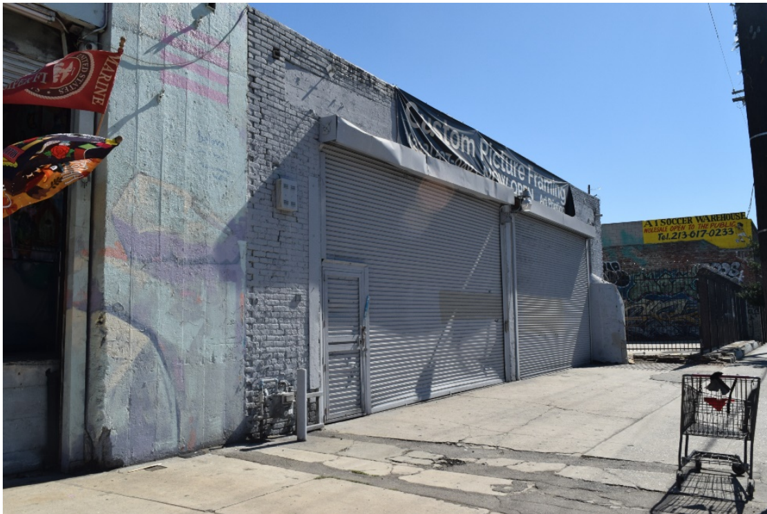
Figure 5-18. 440 South Alameda Street, East Elevation
