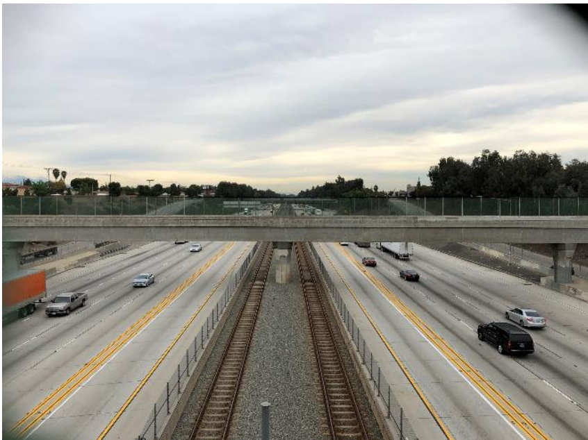
Existing Arthur Avenue Pedestrian Overcrossing
