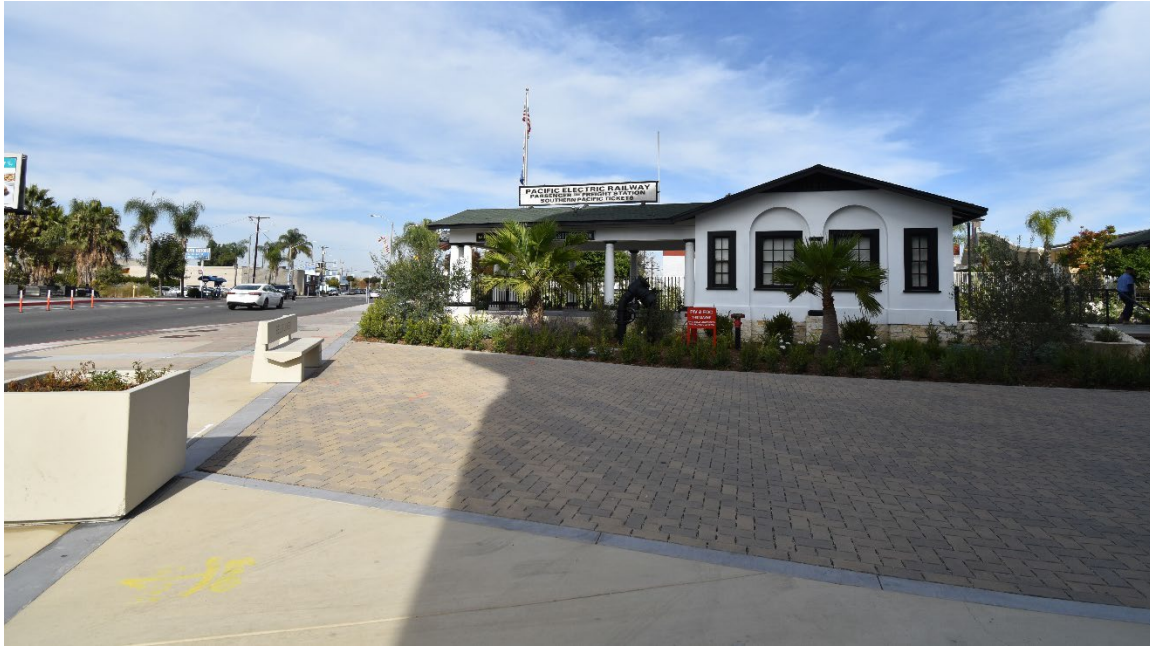
Figure 5-73. Bellflower Pacific Electric Railway Depot, South Elevation
