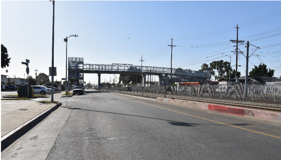
Figure 5-62. Existing 53rd Street Pedestrian Bridge Northeast-Facing
