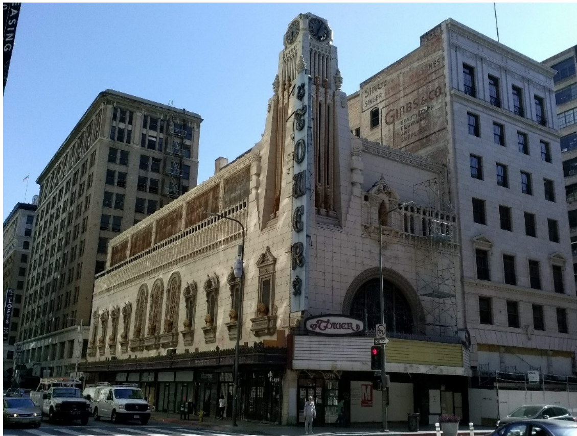
Figure 5-29. 800 South Broadway, North and West (Primary) Elevations
