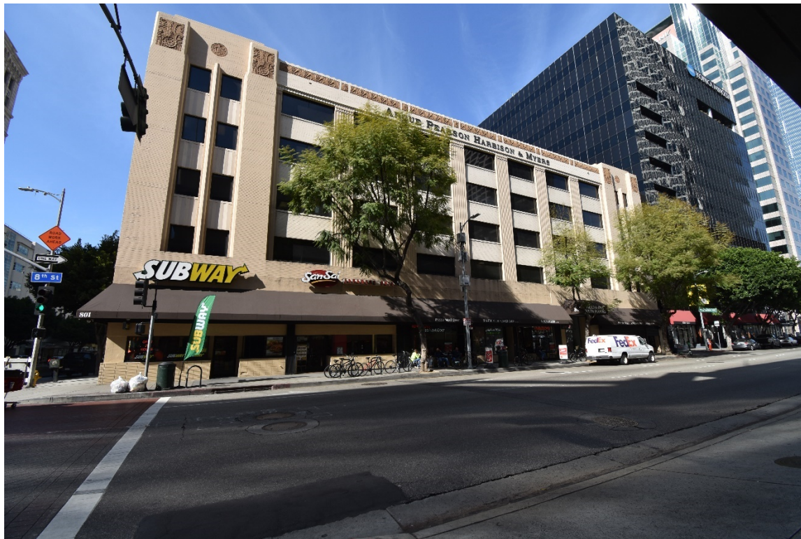
Figure 5-41. 801 South Flower Street, North Elevation
