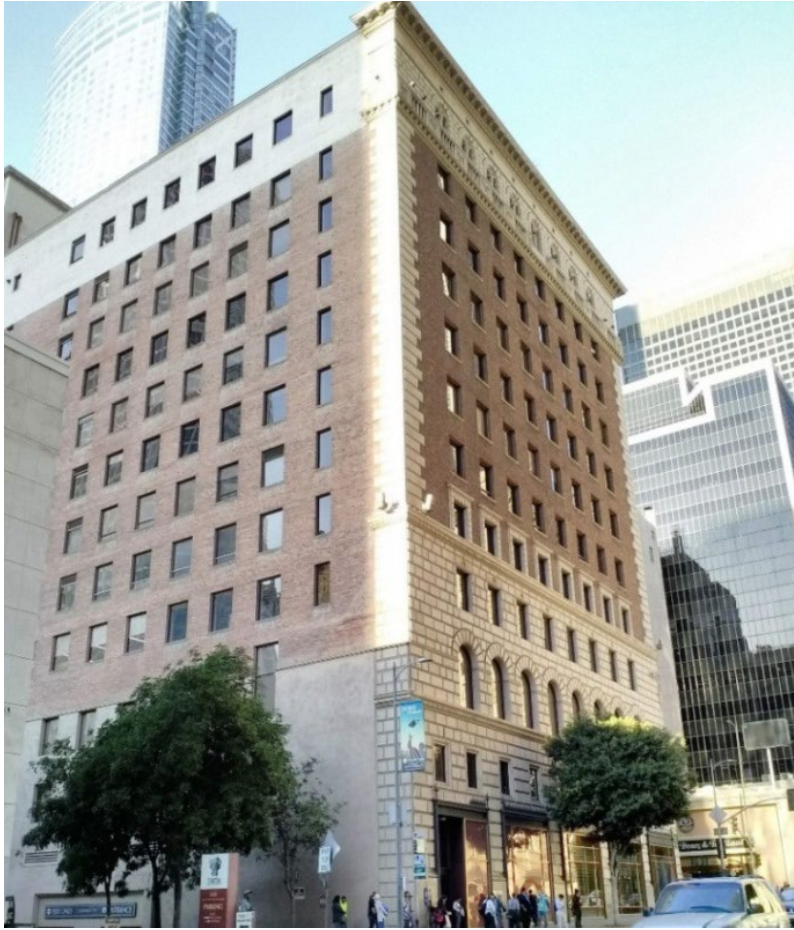
Figure 5-31. Barker Brothers Furniture Store, South and East Elevations
