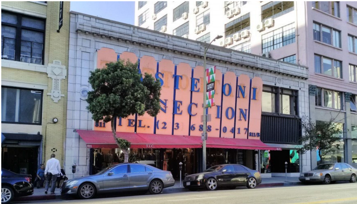
Figure 5-44. 809 South Los Angeles Street, East Elevation
