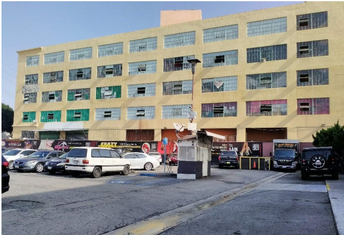
Figure 5-23. 1753 East Olympic Boulevard; Northern-Most Building, South Elevation
