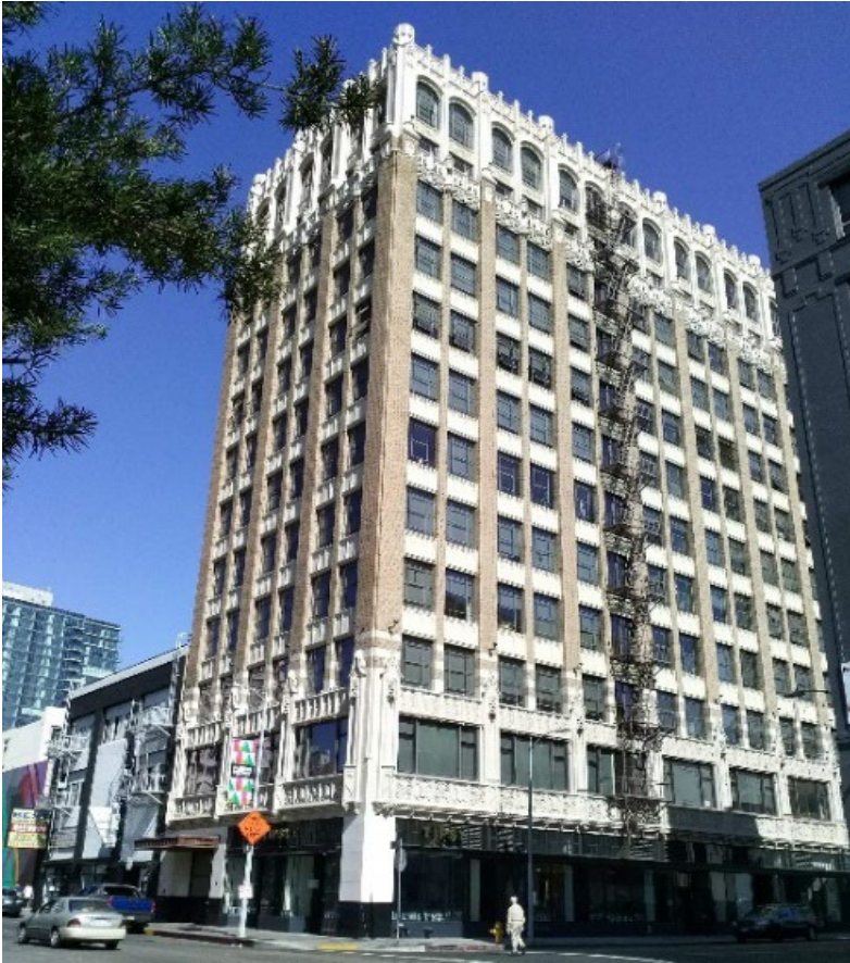
Figure 5-33. Garment Capitol Building, Primary (South and East) Elevations
