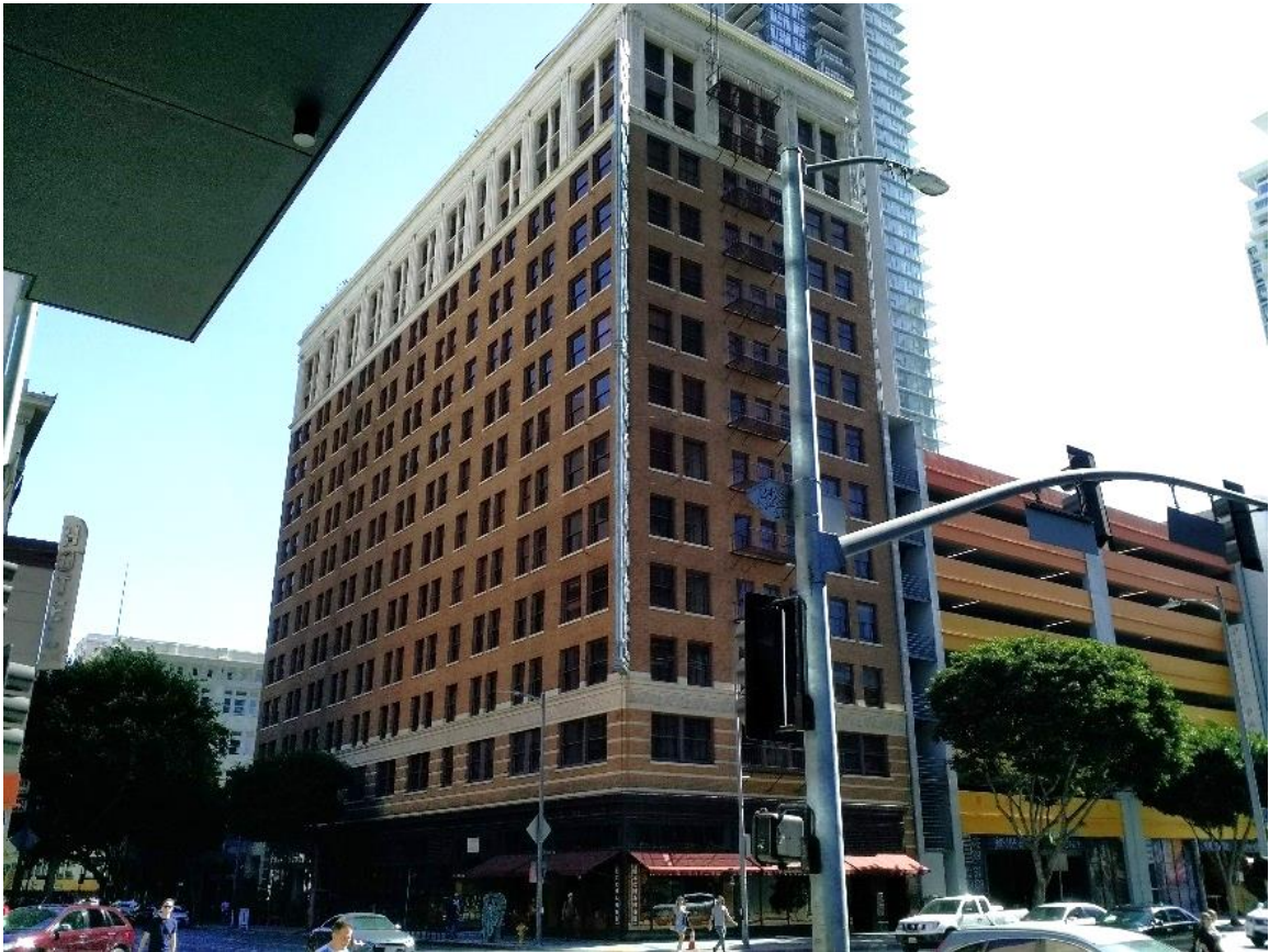
Figure 5-49. Commercial Exchange Building, Primary (North and West) Elevations
