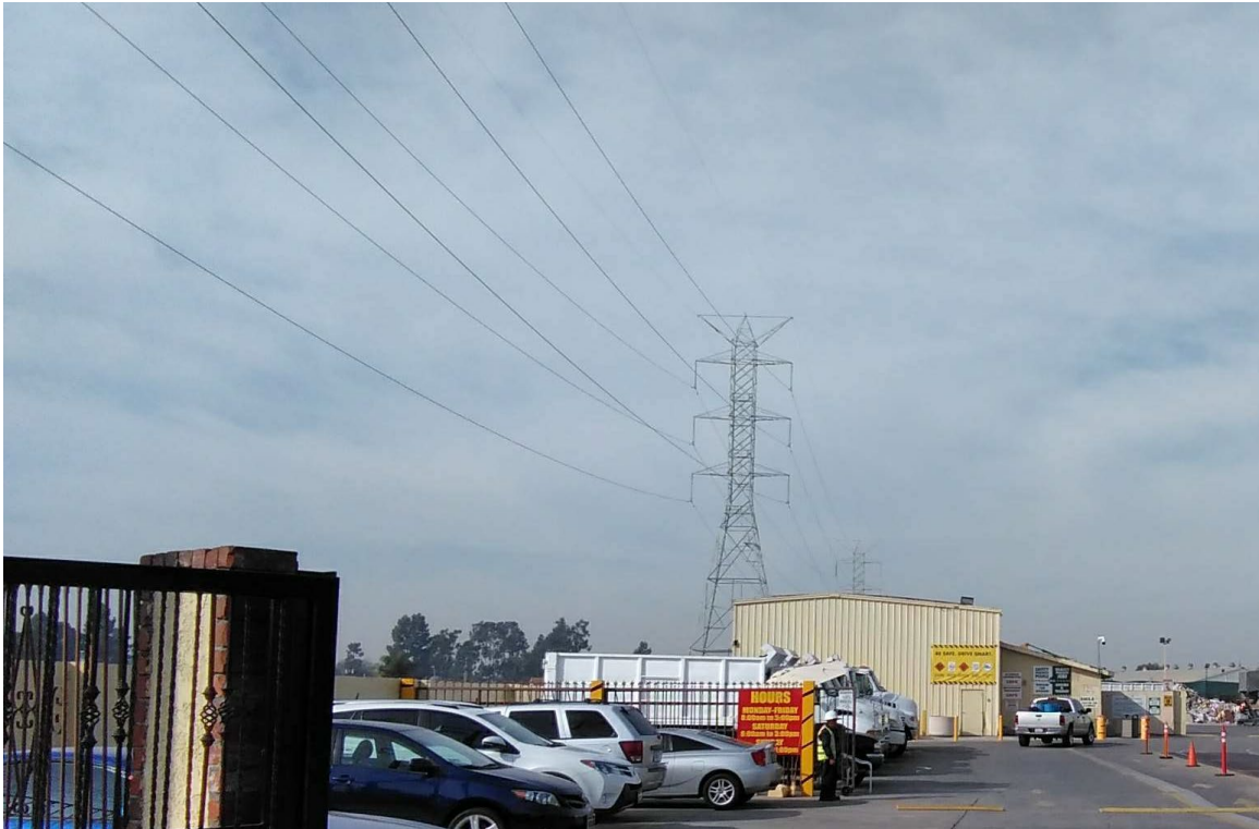
Figure 5-68. LADWP Boulder Lines 1 and 2, Taken near their Intersection with Rayo Avenue, West-Facing
