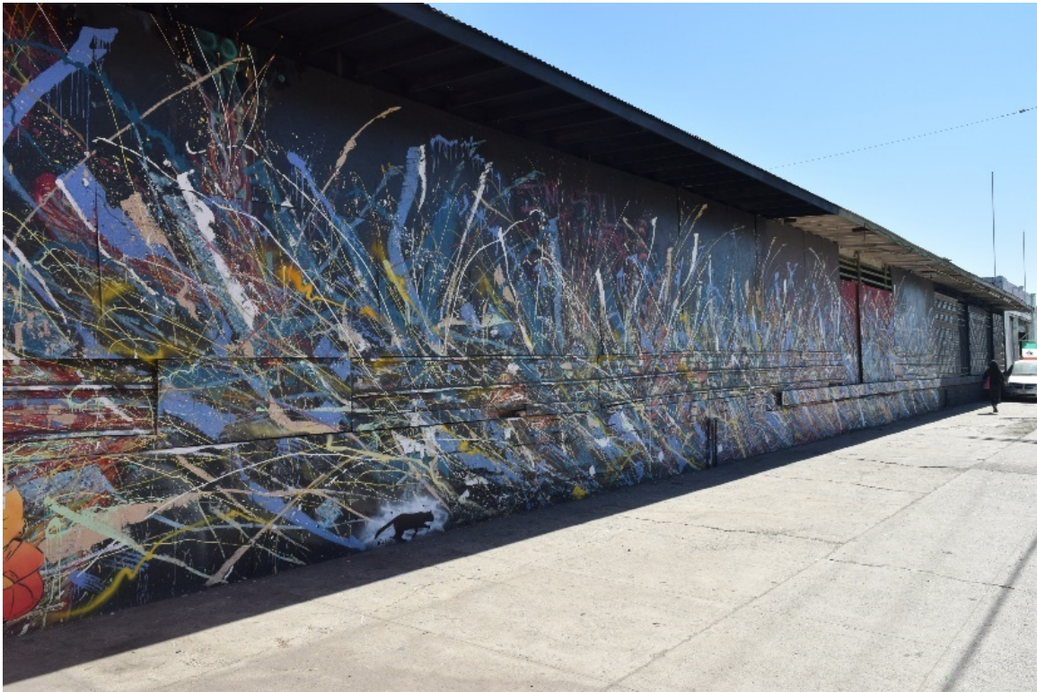
Figure 5-16. 422-430 South Alameda Street, West Elevation
