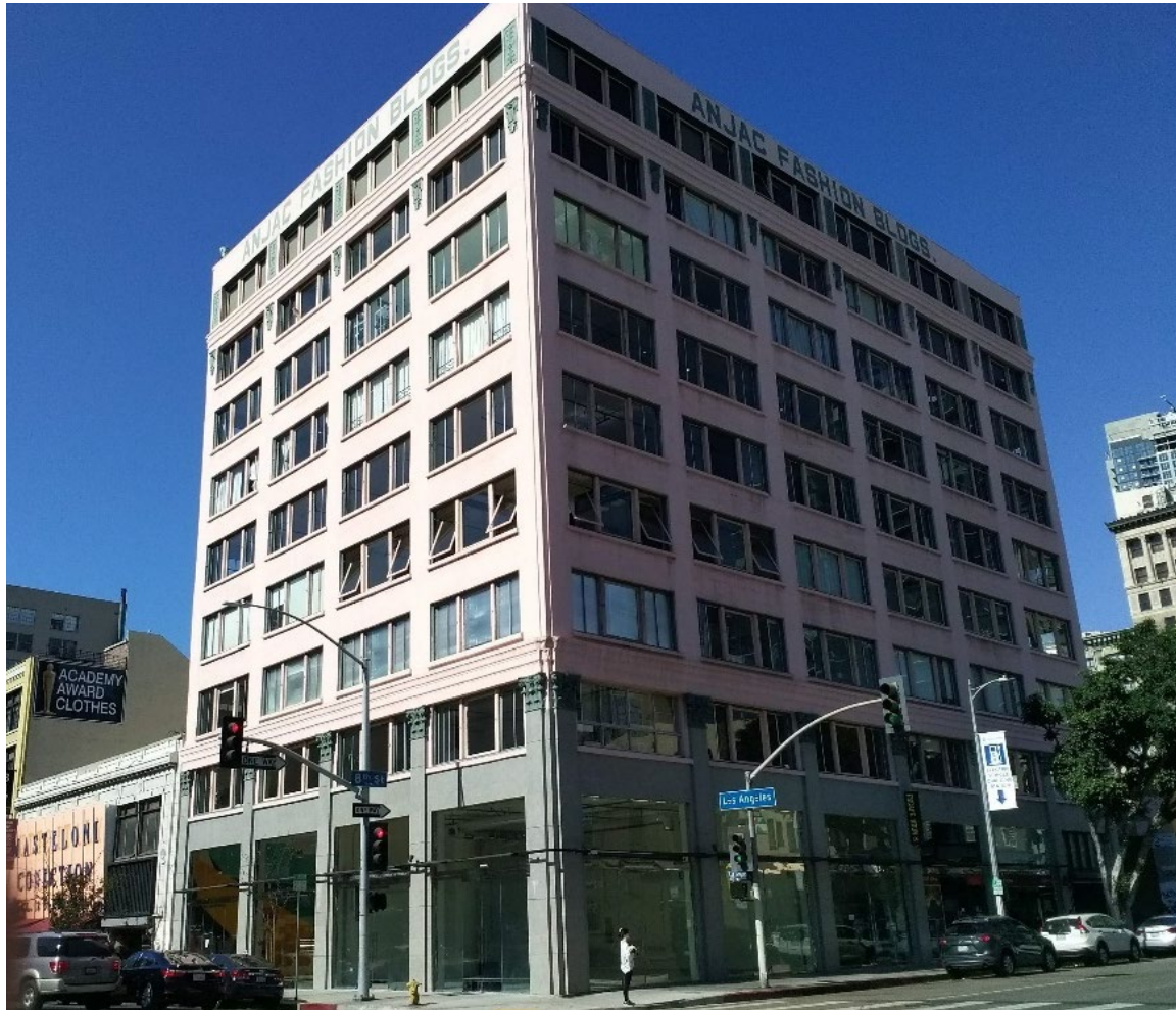
Figure 5-43. 801 South Los Angeles Street, Primary (South and East) Elevations
