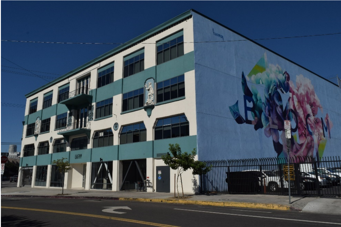
Figure 5-13. 701 East 3rd Street, South and East Elevations
