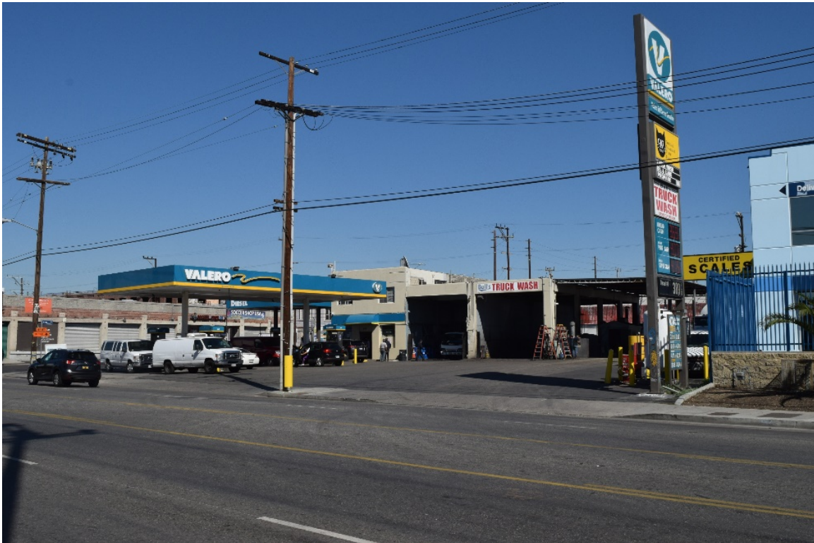
Figure 5-20. 500 South Alameda Street, West Elevation
