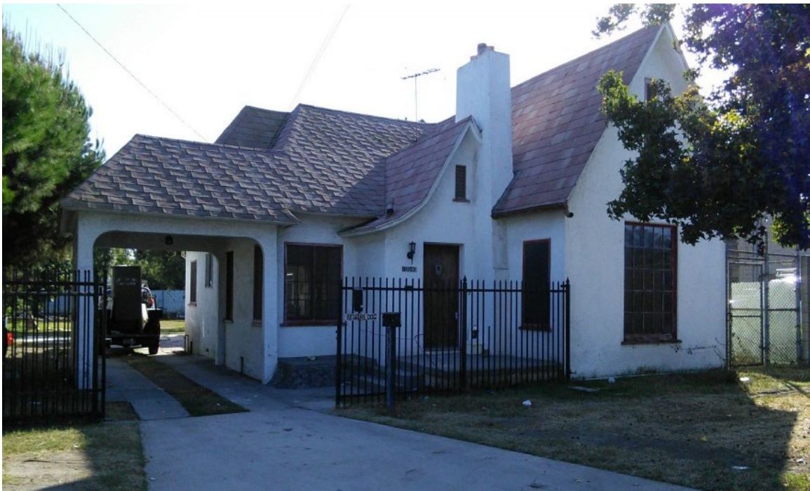
Figure 5-76. 10040 Flora Vista Street North Elevation
