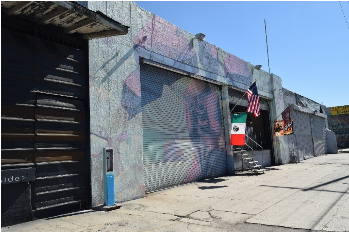
Figure 5-17. 436 South Alameda Street, West Elevation
