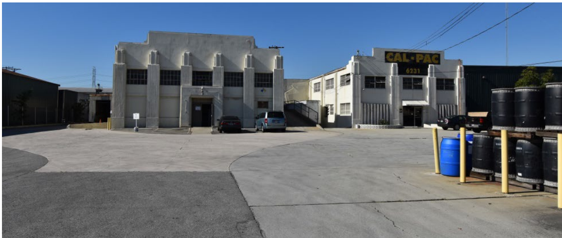
Figure 5-58. 6231 Maywood Avenue, East Elevations
