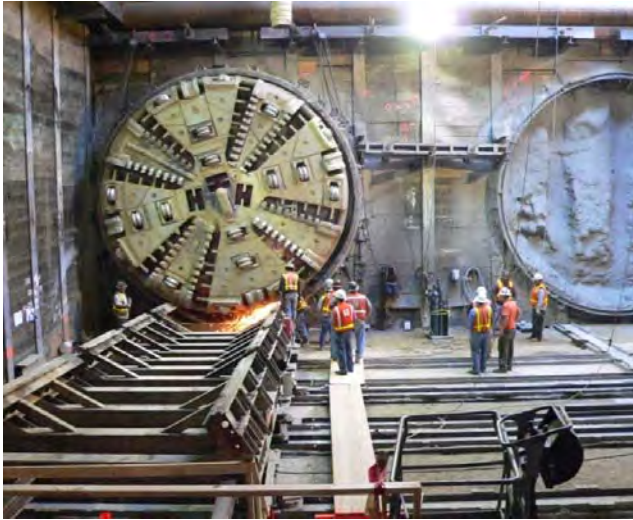
Figure 4-69. Twin Tunnels on Eastside Extension
