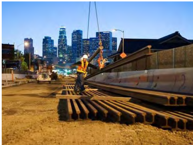
Figure 4-76. Off-Street Construction Area on Metro's Eastside Extension
