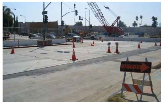
Figure 4-73. Concrete Decking on Street
