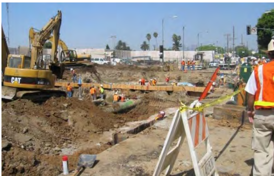
Figure 4-72. Typical Street Excavation
