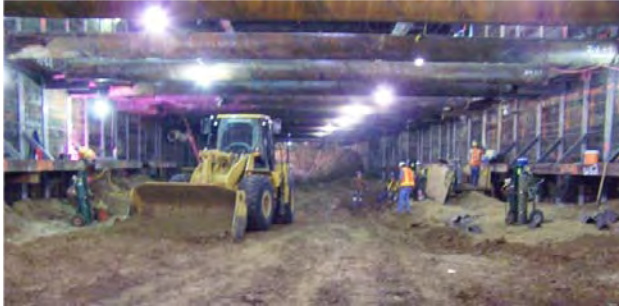
Figure 4-74. Construction Activities below Concrete Decking
