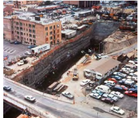
Figure 4-75. Off-Street Station Box Excavation
