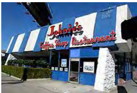
Figure 4-59. Johnie's Coffee Shop Exterior in 2007
