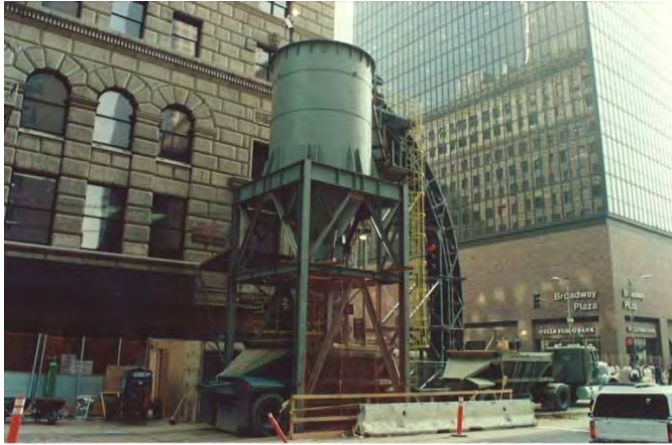
Figure 4-77. On Street Construction Area Used for 7th/Metro Station
