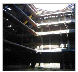
Figure E-5. Typical Soldier Pile and Lagging System (Metro Gold Line Eastside Extension)
