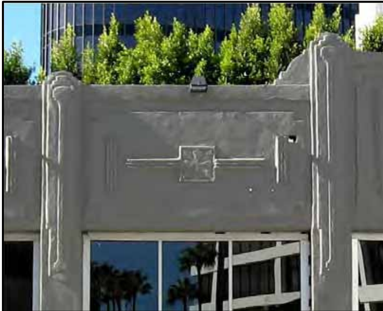
Bas-relief panel over windows on east elevation.
