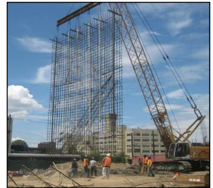
Figure 4-7: Rebar Cage for Typical Slurry Wall Panel
