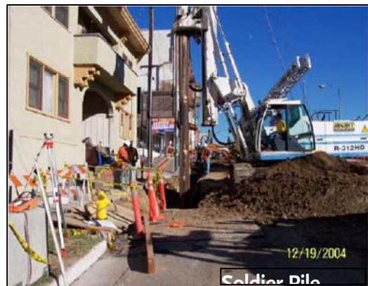
Figure 4-3: Drilling for Soldier Pile Installation
