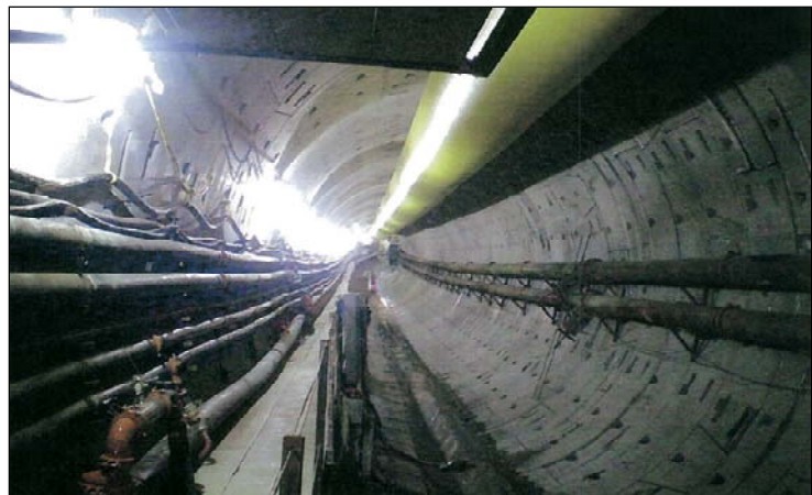
Figure 4-18: Typical TBM Tunnel Shown During Construction
