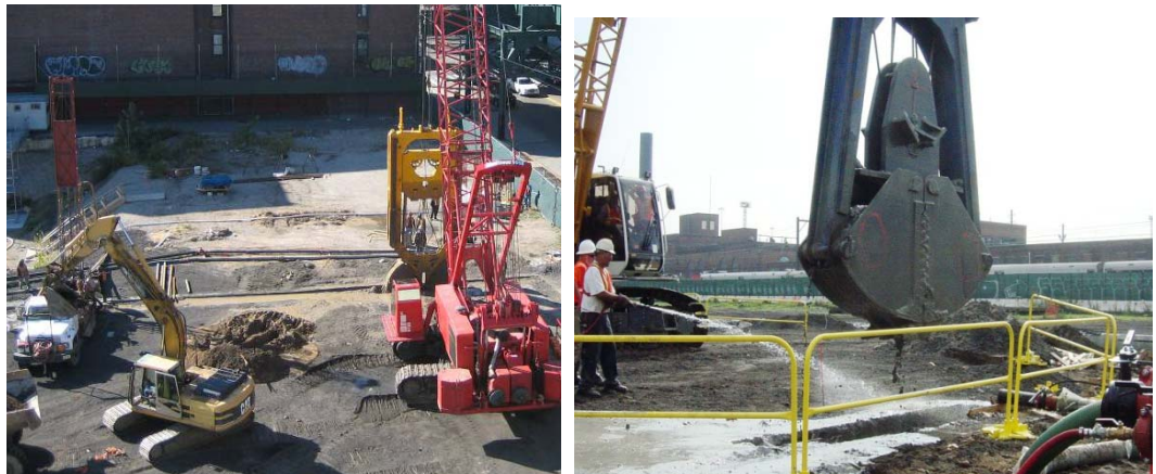
Figure 4-6: Typical Slurry Wall Panel Excavation
