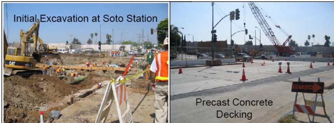
Figure 4-2: Typical Cut-and-Cover Construction Activities from the Metro Gold Line Eastside Extension
