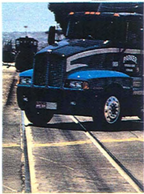
Present Condition At-Grade Highway Crossing
