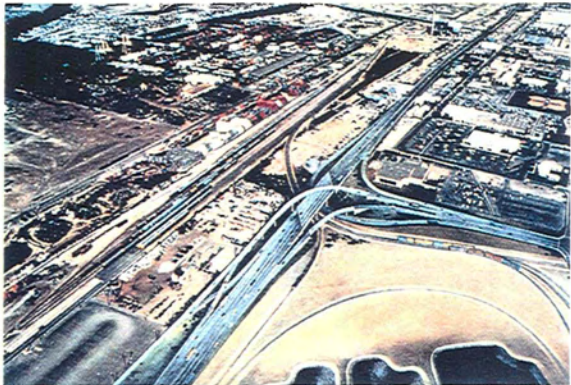
Cross Street Grade Separation
