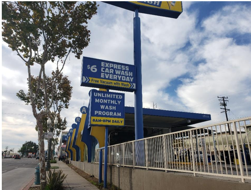
Figure 3.13-10. Overview of 17101 Hawthorne Blvd. property, view to southwest, November 5, 2020
