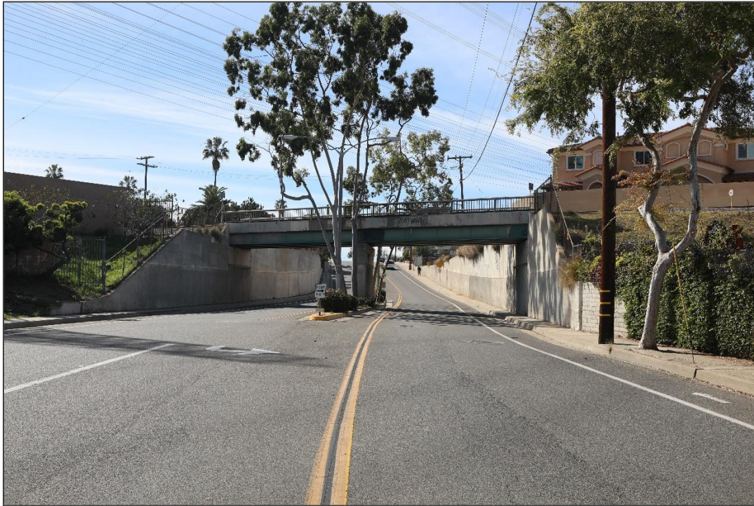
Figure 3.3-64. KOP 8 – Before and After Simulation View, View looking west from Grant Avenue towards the Proposed Project Relocated Freight Bridge and Elevated Alignment
