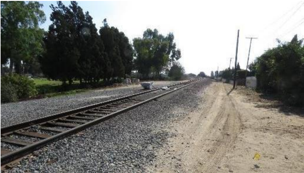
Figure 3.7-7. Metro ROW with current freight track, south of 182nd Street; facing south
