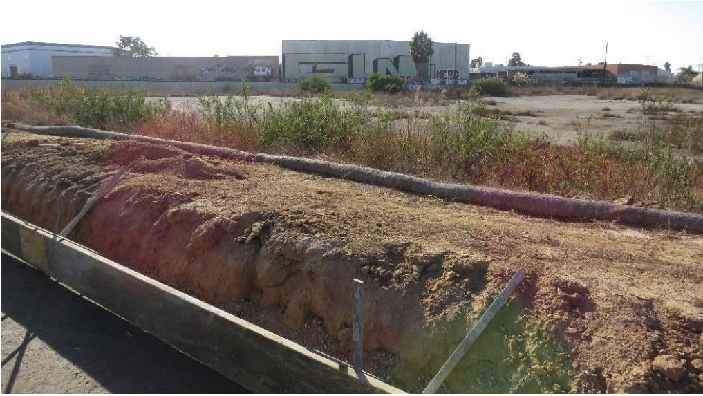
Figure 3.7-6. View Across Torrance TC Towards Proposed Station at Torrance TC; facing southwest
