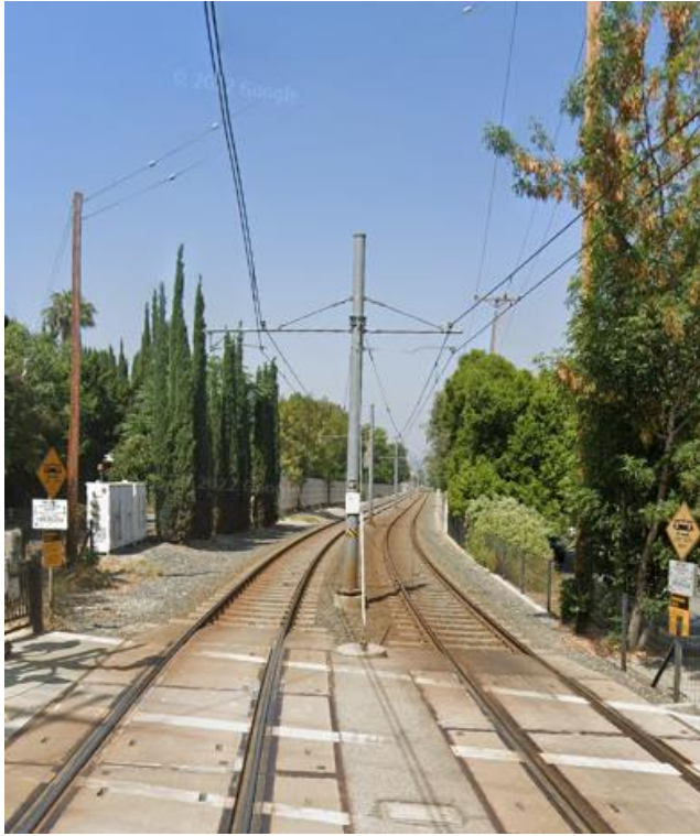
Figure 2.3-32. Typical OCS
