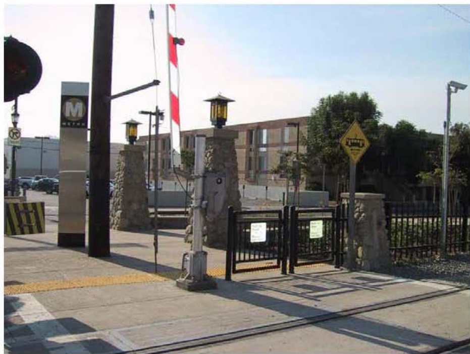
Figure 3.12-1. At-Grade Light Rail Transit Crossing with Safety Features
