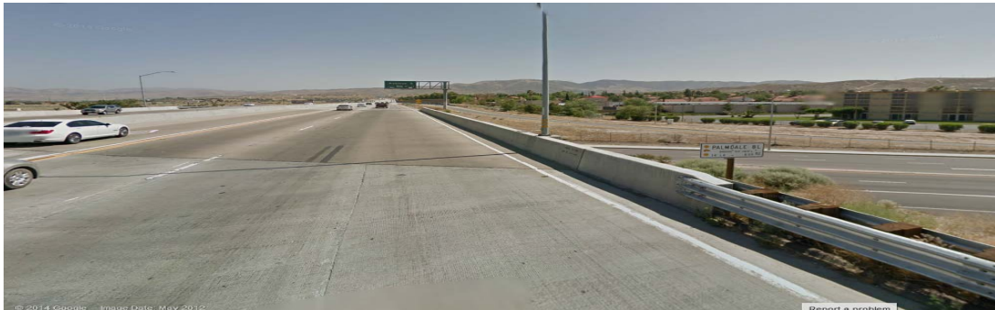
Figure 3.1.7-7 KV #2 Existing View
