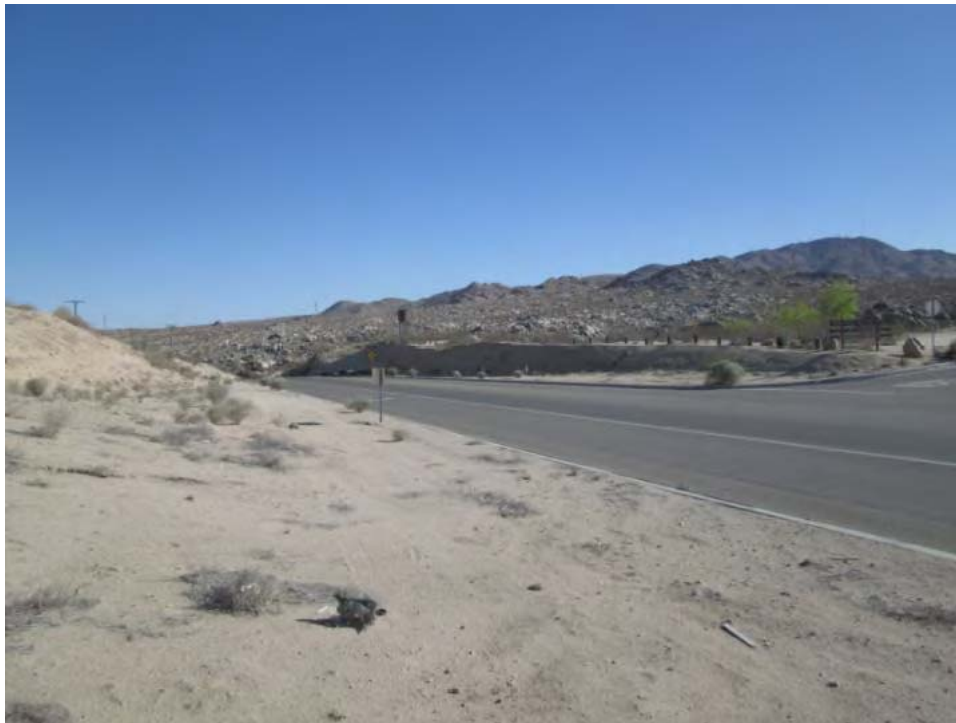
View looking north at segment of National Old Trails Highway/Route 66 in the APE. Rockview Nature Park is to the right (east side of the road).
