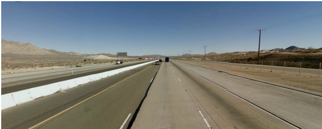
Figure 3.1.7-48 KV #21 Existing View
