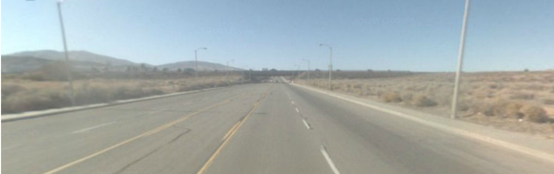
Figure 3.1.7-18 KV #6 Existing View
