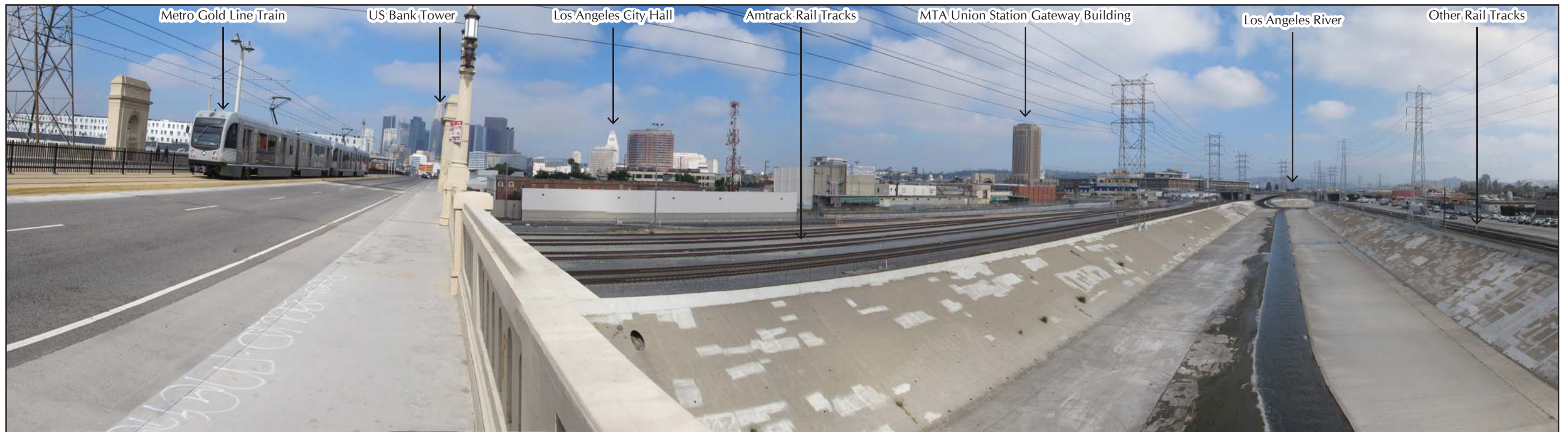
PHOTO 8. E 1st Street Bridge Over Los Angeles River in April 2016 - Facing North
