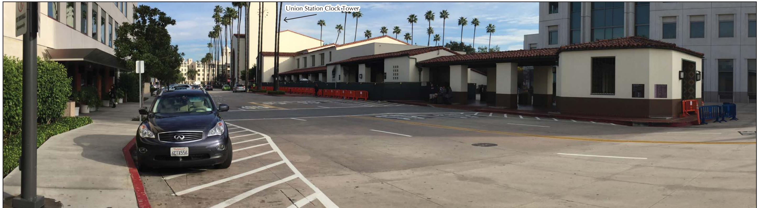
PHOTO 16. Sidewalk Adjacent to First 5 LA Building in February 2017 – Facing Northeast
