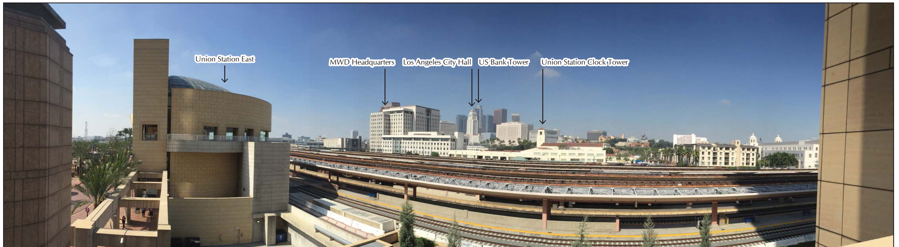
PHOTO 10. MTA Union Station Gateway Building at Union Station East in April 2016 – 3rd Floor Balcony – Facing Southwest
