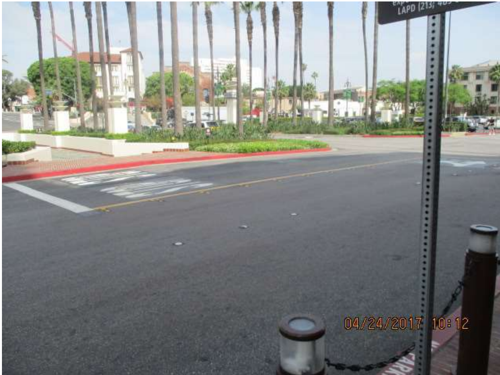
Photograph 8 - View facing northwest at the LAUS entrance and forecourt area of the Project.
