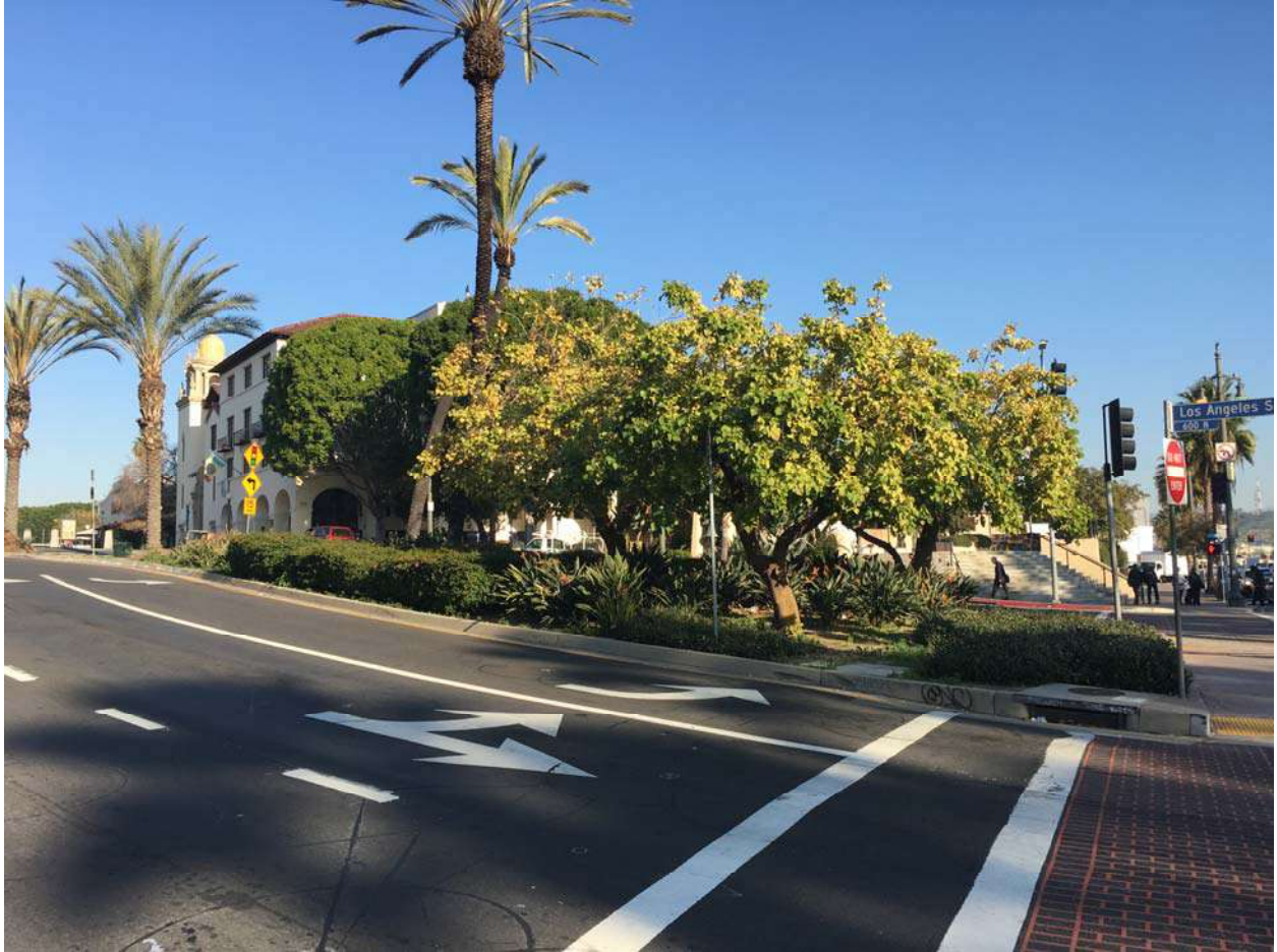
FIGURE 6.2-2 Southwest Corner of Los Angeles St. and Alameda St., View to North
