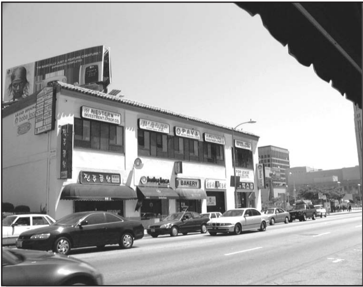
Retail/office building on Western Avenue to be demolished.
