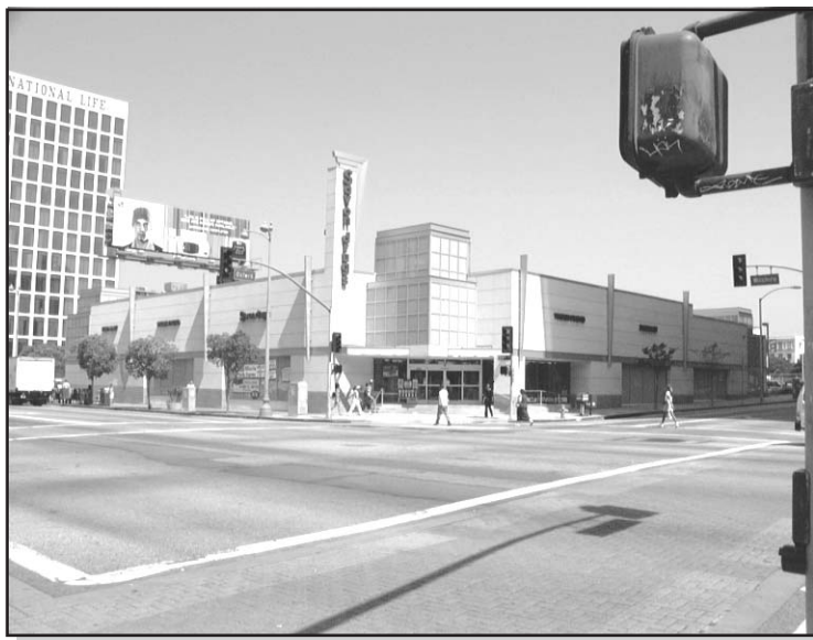
Retail building to remain which is located along the south/east boundary of the proposed project site.
