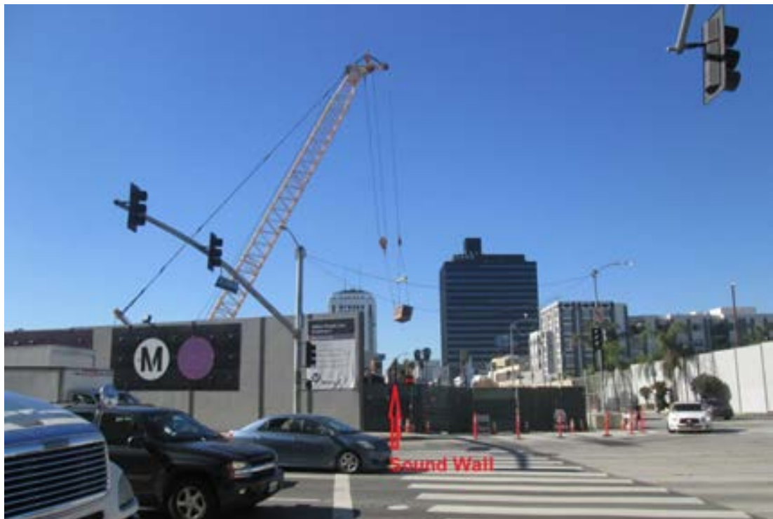
Figure 4-29. Crane at the Wilshire/La Brea Muck Shaft
