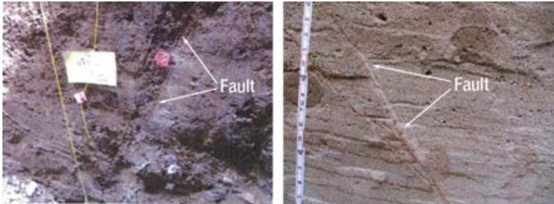
Figure 4-35. Photographs of faults encountered in trench explorations (a) at BHHS (LCI, 2012a), and (b) Newport-Inglewood Fault at Los Angeles Southwest College (Mactec, 2007)
