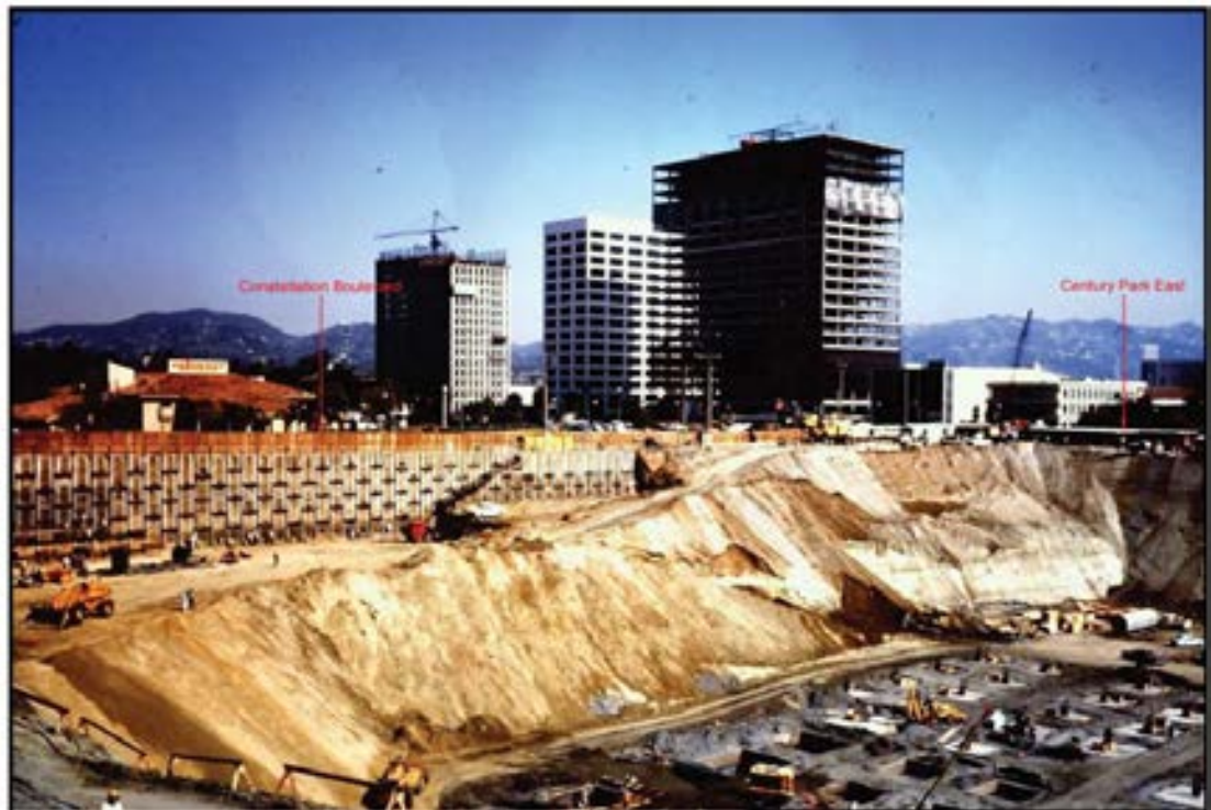
Figure 4-11. Century City Theme Towers during Construction circa 1972 – North Side of Excavation Illustrating Lack of Faulting in Soil Layers
