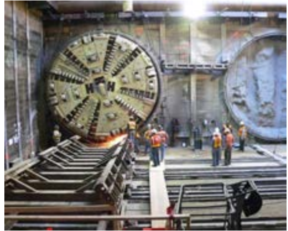
Figure 4-23. Twin Tunnels on Eastside Extension
