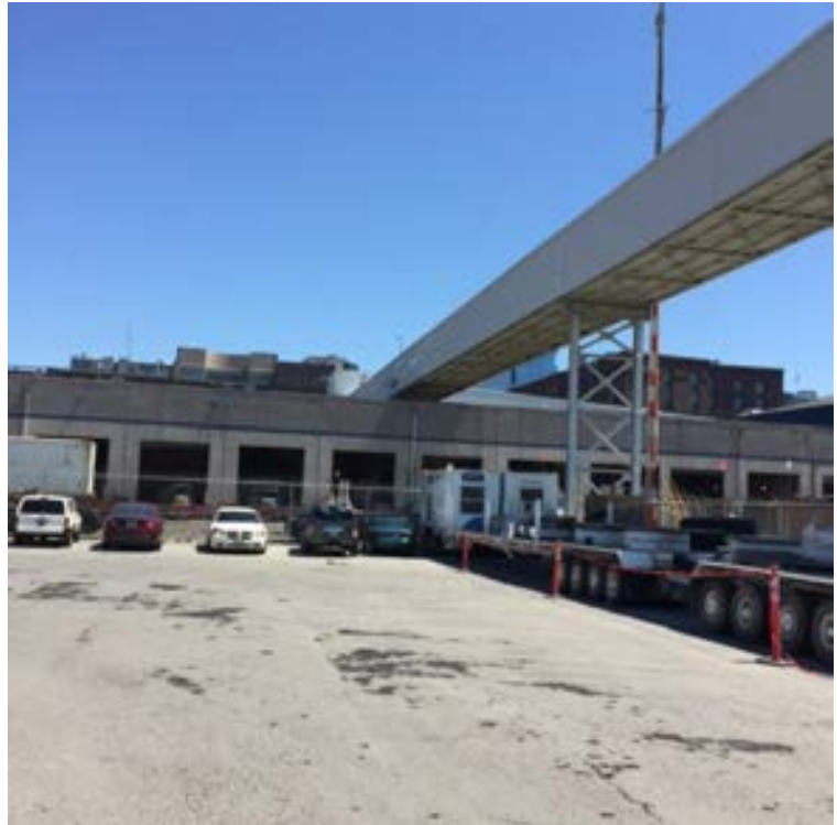
Figure 4-30. Typical Enclosed Conveyor
