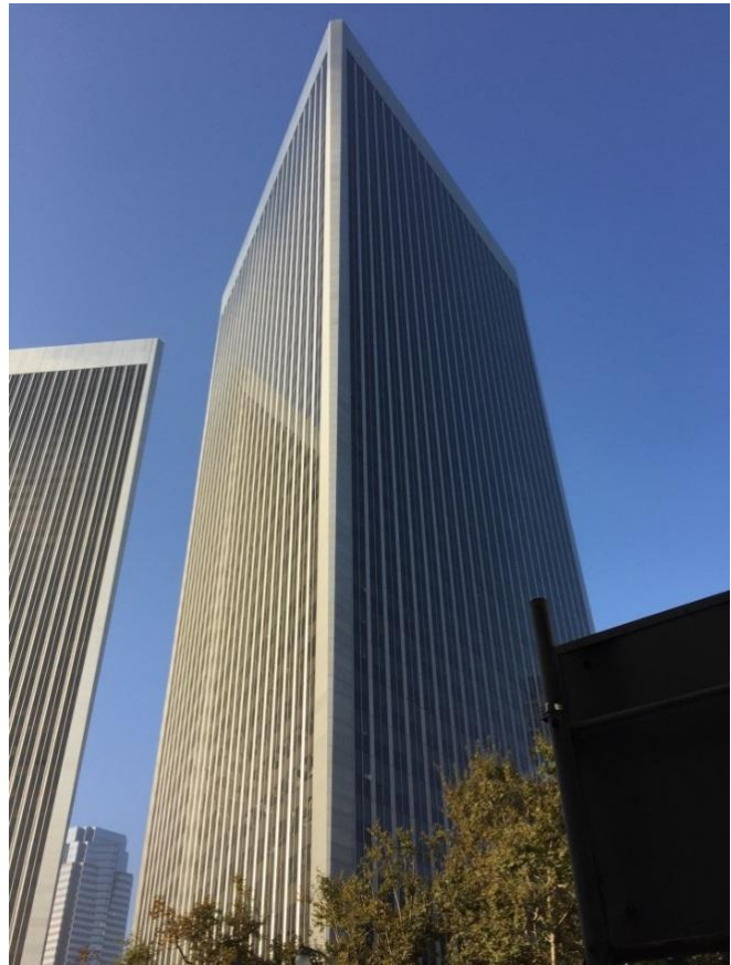
Figure 5-9. Century Plaza Tower
