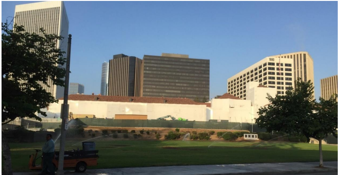
BHHS, under renovation August 2016
