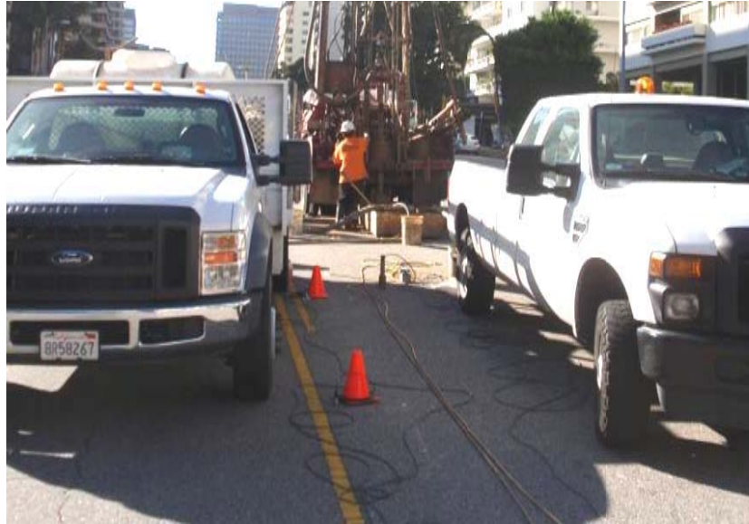
Figure 62: G-178 Wilshire/Manning. View looking west along Wilshire Blvd.
