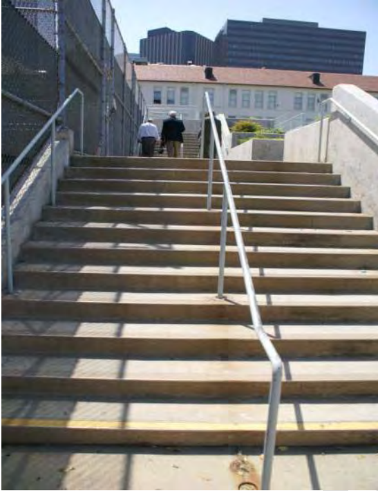
Figure C-7: Pathway leading to Building B
