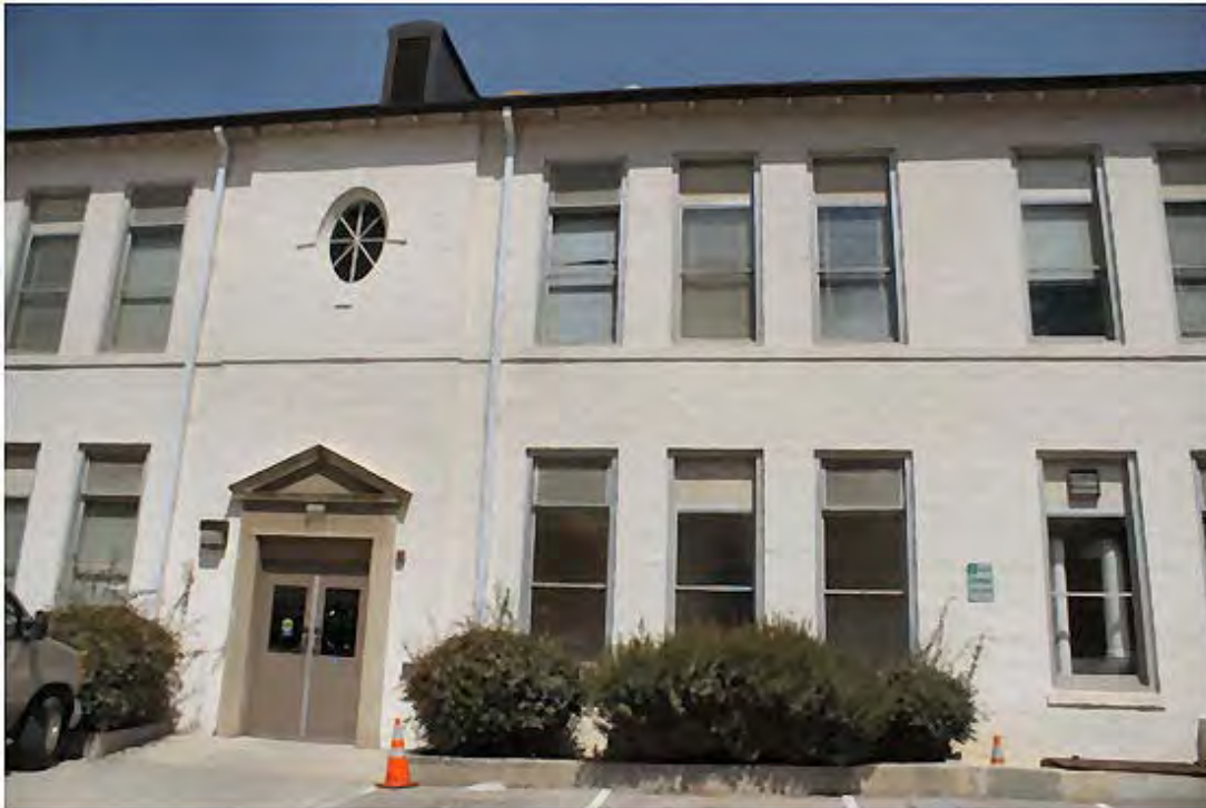
Figure C-11: Building B—Exterior Looking West
