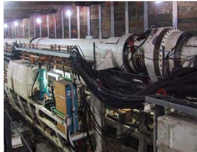
Figure 5-6: EPBM Screw Conveyor for MGLEE
