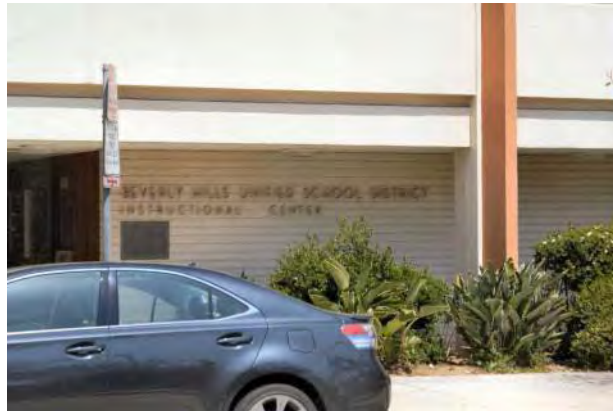
Figure C-2: Instructional Center Building
