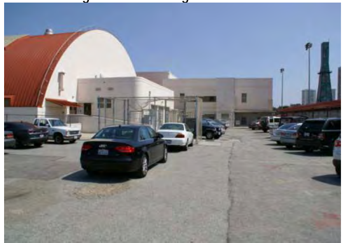
Figure C-6: Building F—Arch Roof
