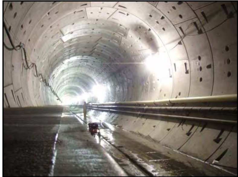
Figure 5-9: Segmental Lining
