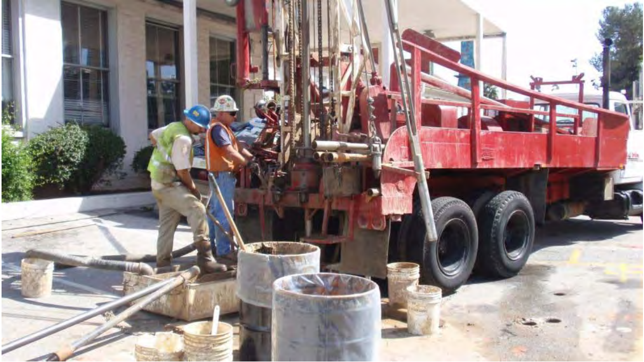
Figure 8-3: Drill Rig Outside BHHS Classroom Building
