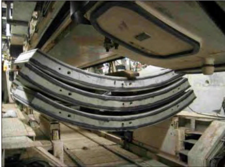
Figure 5-5: Double-Gasketed Segments at Tunnel Heading
