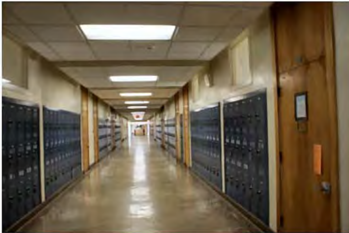
Figure C-9: Building B—Interior Corridor
