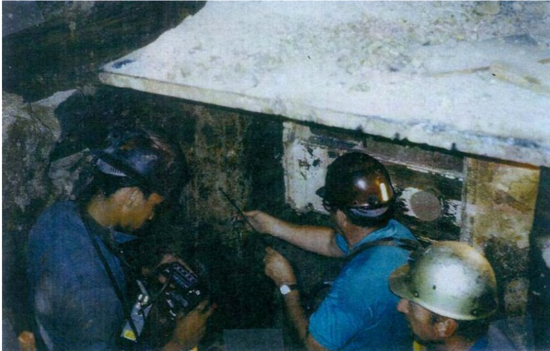
Figure 6-9: Probing of Oil Well Casing, Metro Red Line, Downtown Los Angeles
