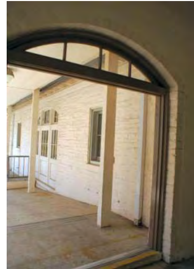
Figure C-10: Building B Interior
