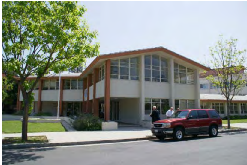
Figure C-1: Administration Building—Steel Framed Structure—Built in 1960s
