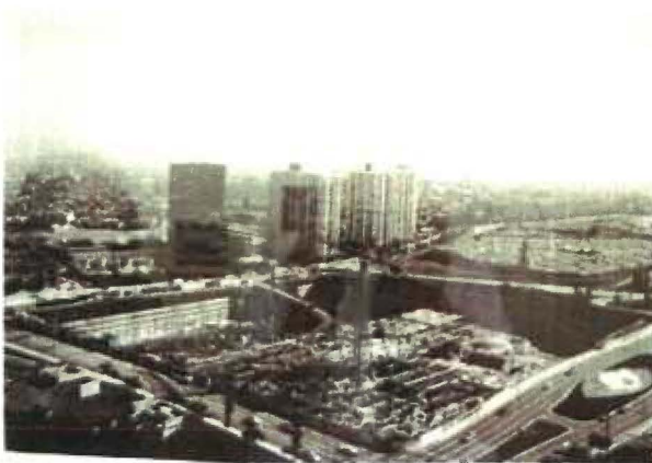
Underground Construction Constellation Boulevard
