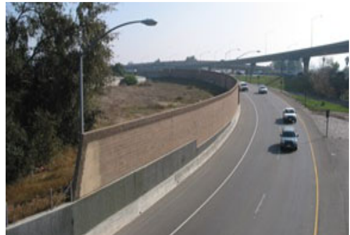
Typical Noise Barrier Along a Freeway
