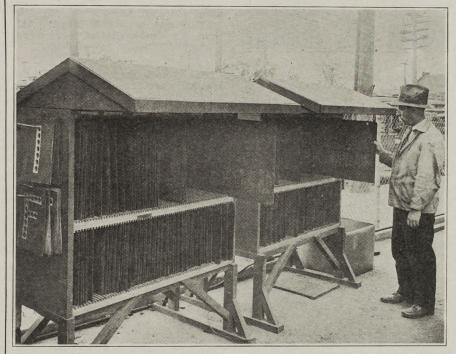
FTER a test of several months, the new type of rack for holding the metal dash signs at the car house, has proved its superiority over the holders formerly used and has reduced the work of painting and lettering the signs considerably.
