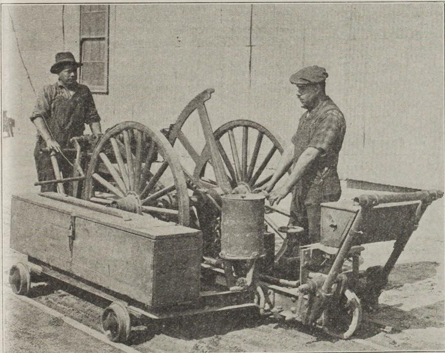
ALTHOUGH it looks somewhat like a cross between a lawn-mower and a Ford, the reciprocating rail grinder used by the track department is one of the most valuable pieces of machinery for the convenience of riders. The track grinder is used to smooth joints and other parts of track to provide a uniform level and to avoid a drop from one section of rail to another.
