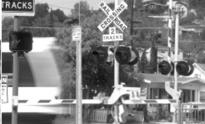
Four-quadrant gates, which have prevented car versus train accidents on the Metro Blue Line, have been installed at key Metro Gold Line intersections.
