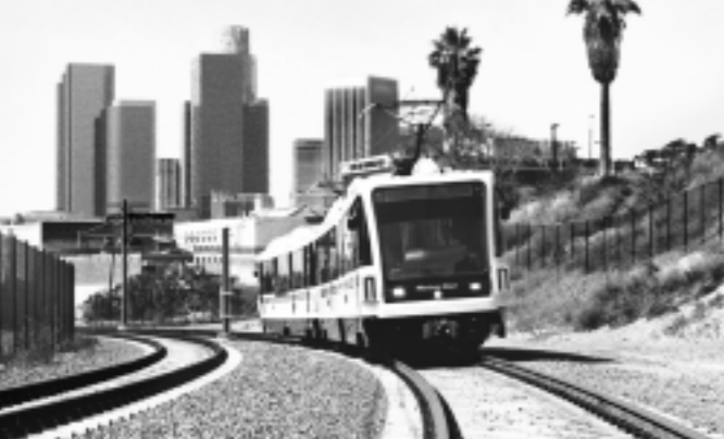
Shortly after departing the Chinatown Metro Rail Station, a northbound Metro Gold Line train is just minutes away from its next stop, the Metro Rail Lincoln Heights/Cypress Park Station.
