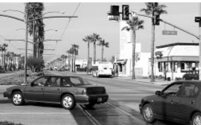
Metro is installing left-hand turn warning signals along Metro Blue Line in Long Beach to improve safety.
