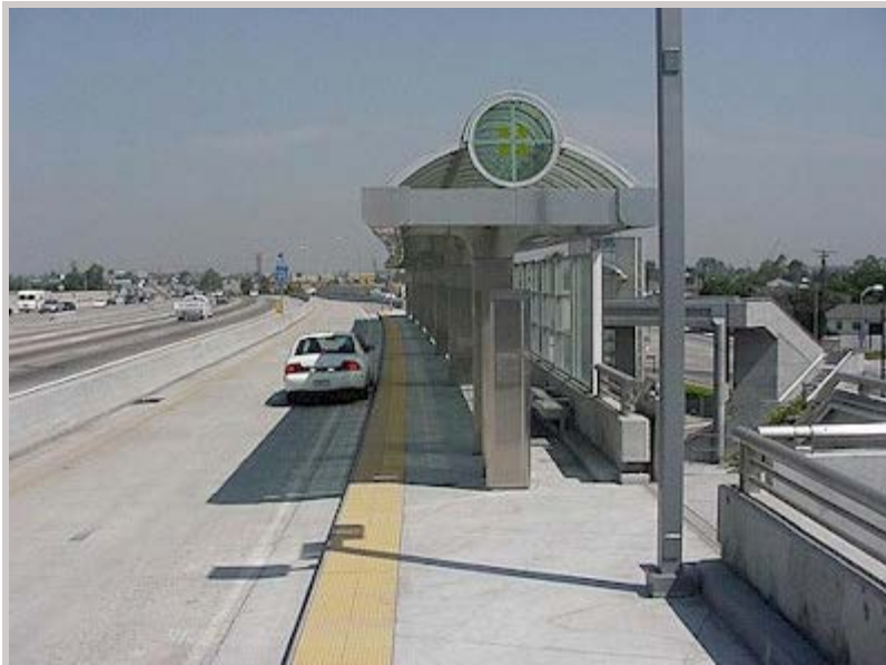
THE BUS STOPS HERE - Northbound Pacific Coast Highway Station is one of two new bus stations opening Sunday along the Harbor Transitway. PHOTO BY JOSÉ UBALDO
