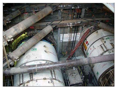
Creating a 21-foot, 4-inch-wide tunnel under East Los Angeles will be no sweat for "Lola" and "Vikki," two German-manufactured tunnel boring machines. The machines will excavate the dirt and process it through to the back of their 344-foot bodies, while also installing the 8,000-pound concrete tunnel liner segments as they go. At \$10 million each, "Lola" and "Vikki" are a fraction of the \$898.8 million cost for the entire Gold Line Eastside Extension. (2/24/06)
