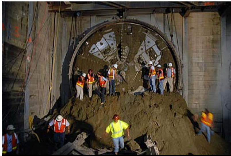
Construction crew claims victory.
