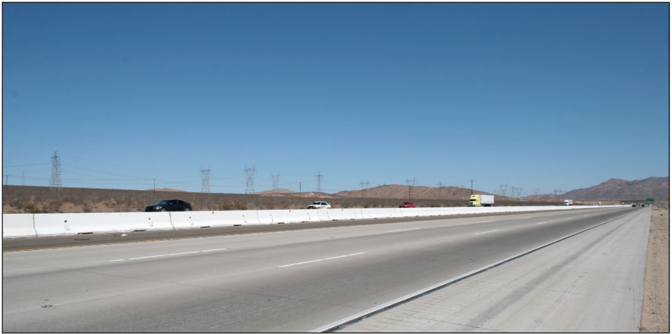
Existing view from I-15 eastbound
