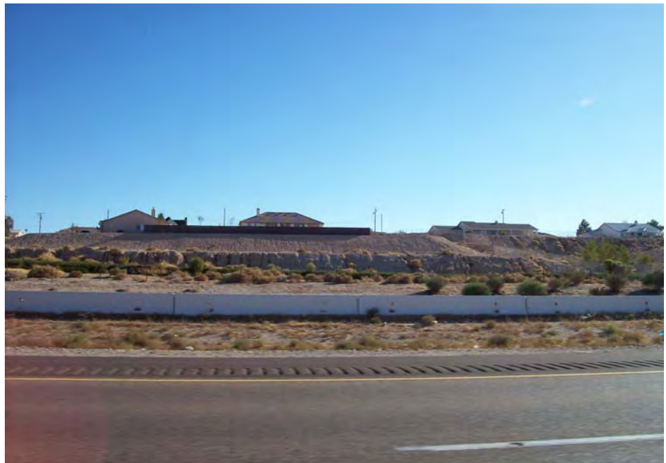
Photograph No. 8: Looking south at the I-15 median and residential properties in Barstow, California.
