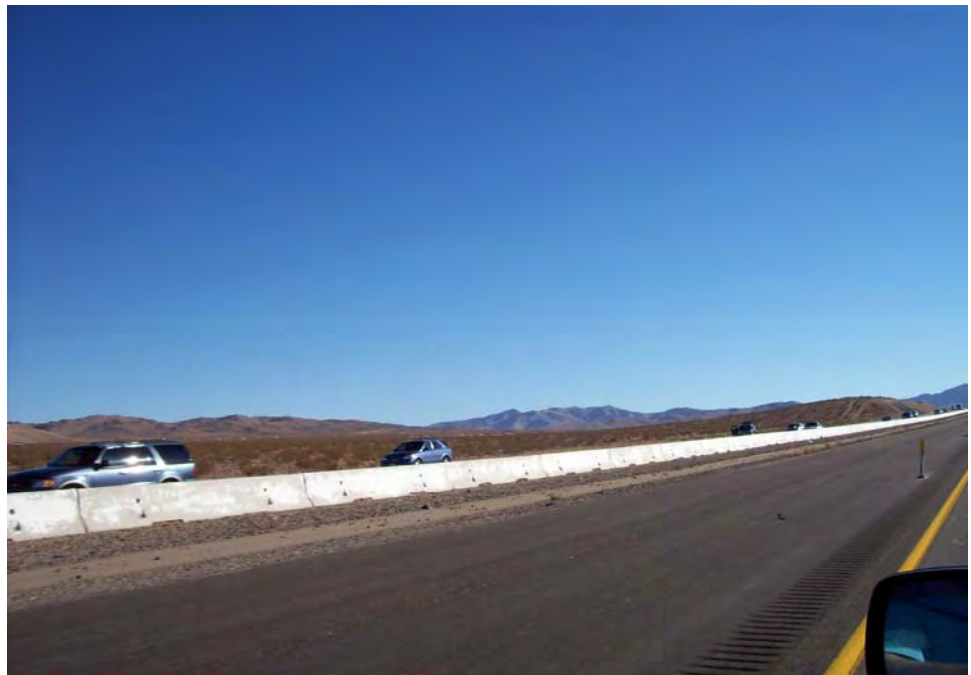
Photograph No. 16: Looking southwest at the southbound I-15 median, south of Lenwood, California.
