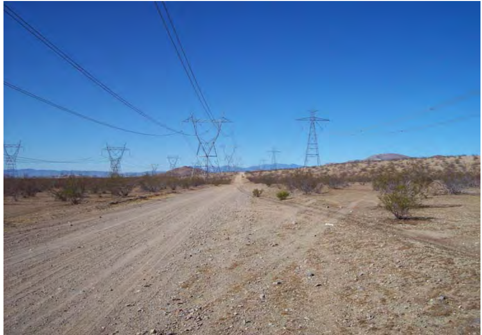
Photograph No. 1: Looking south from Dale Evans Parkway at the proposed Victorville 3 Station area.
