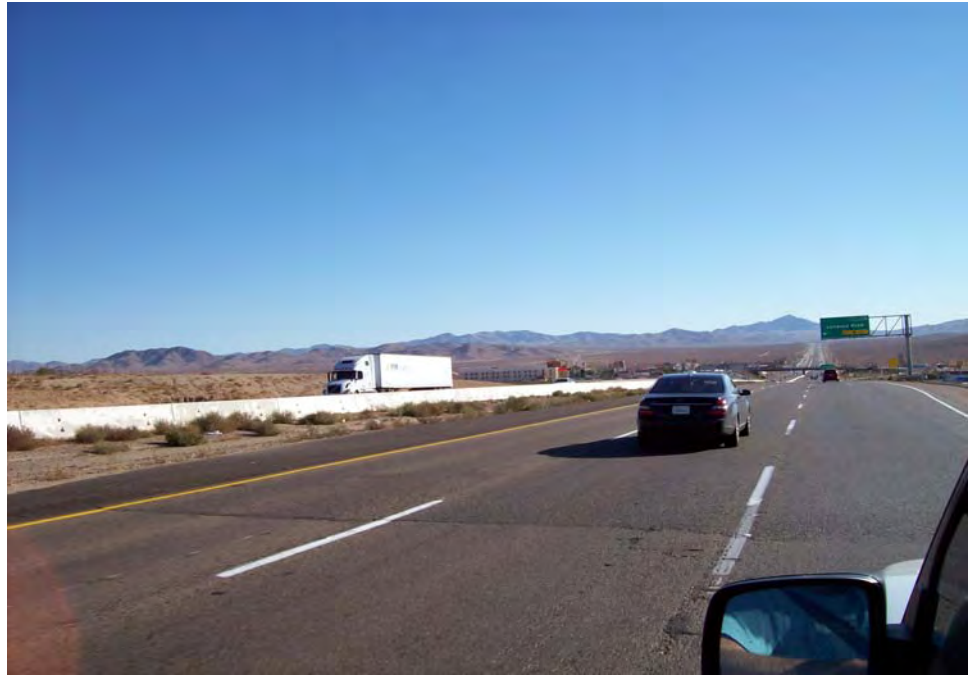
Photograph No. 11: Looking south at southbound I-15 just north of Lenwood, California.
