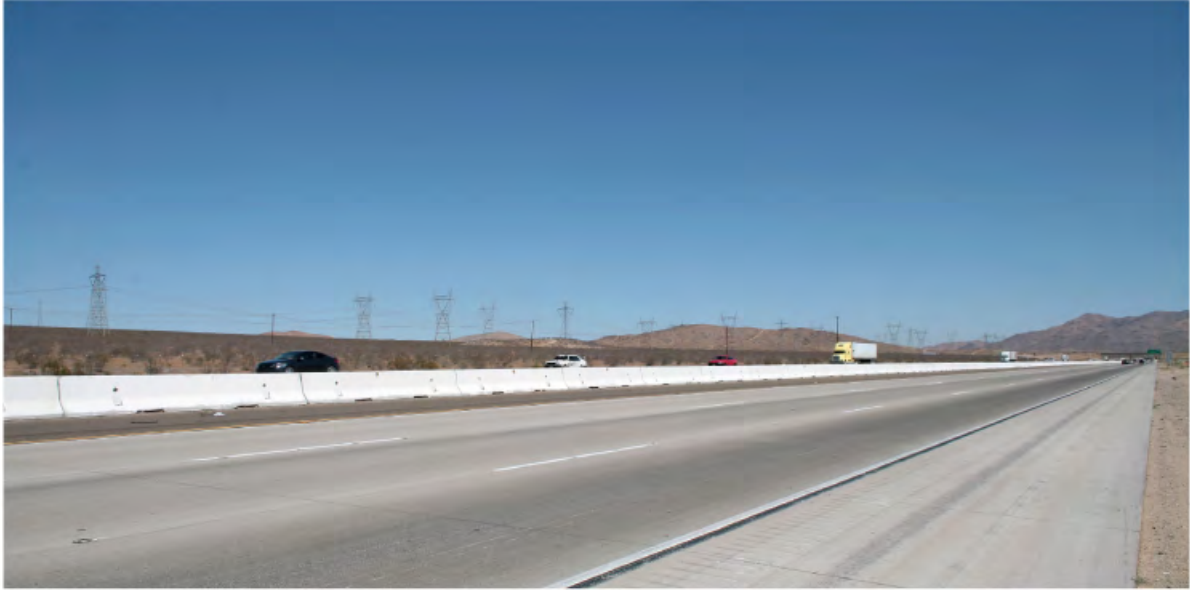
Existing view from I-15 eastbound
