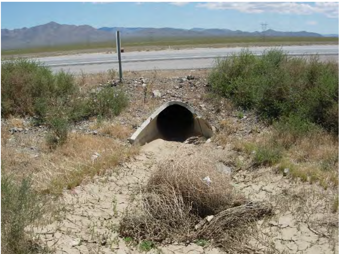
Exhibit A. Figure 16. Manmade drainage connecting to road culvert within HUC 8 Ivanpah-Pahrump Valleys Watersheds / HUC 12 Ivanpah Subwatershed
