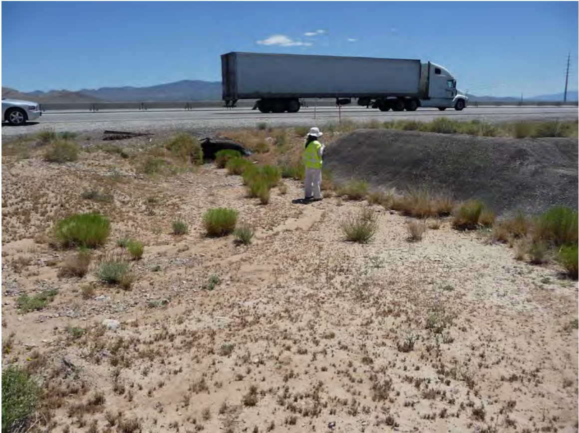
Exhibit A. Figure 35. Manmade drainage connecting to road culvert within HUC 8 Ivanpah-Pahrump Valleys Watersheds / HUC 12 Town of Jean -Frontal Ivanpah Lake Subwatershed
