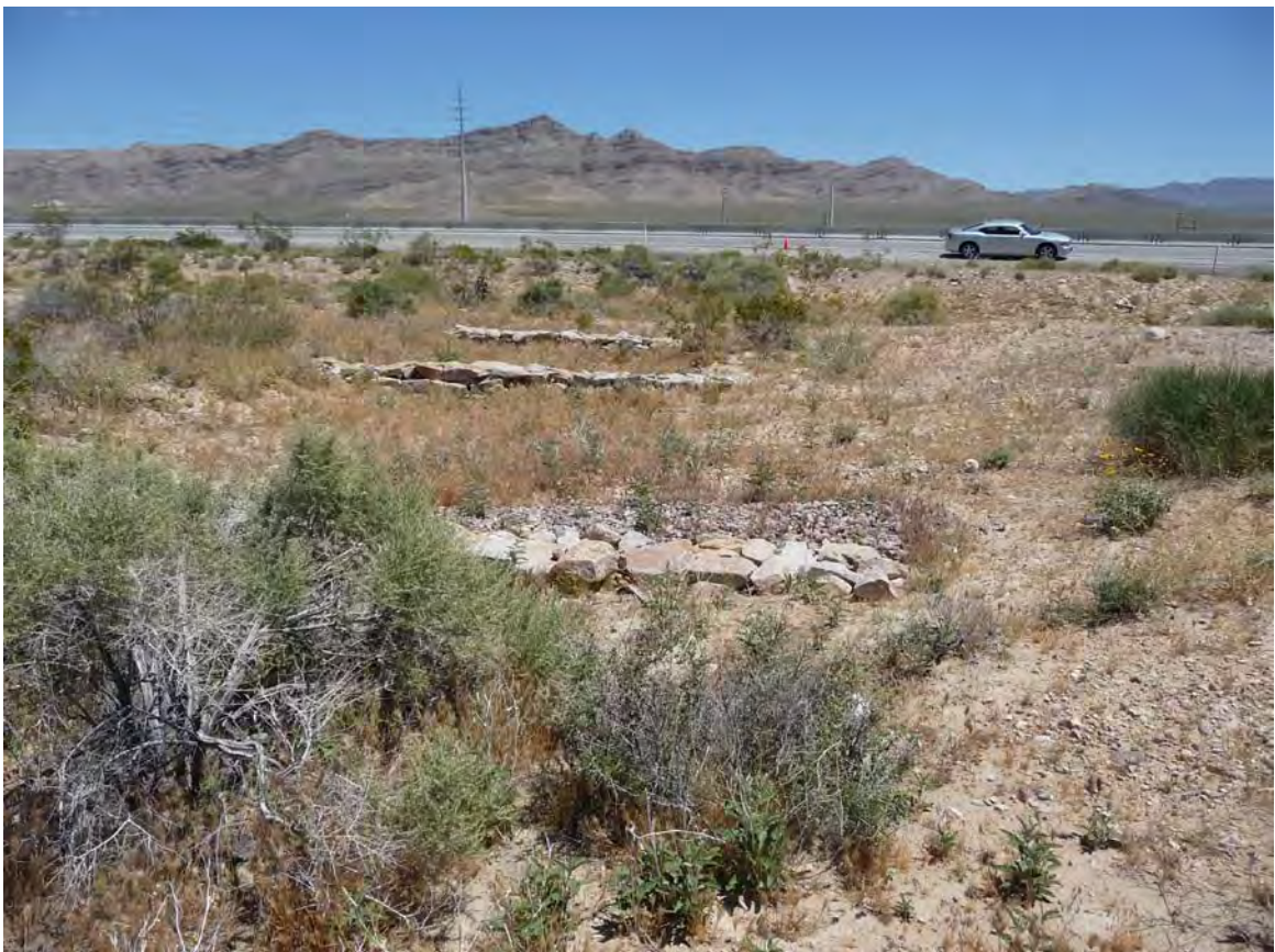
Exhibit A. Figure 36. Manmade drainage connecting to road culvert within HUC 8 Ivanpah-Pahrump Valleys / HUC 12 Town of Goodsprings Subwatershed
