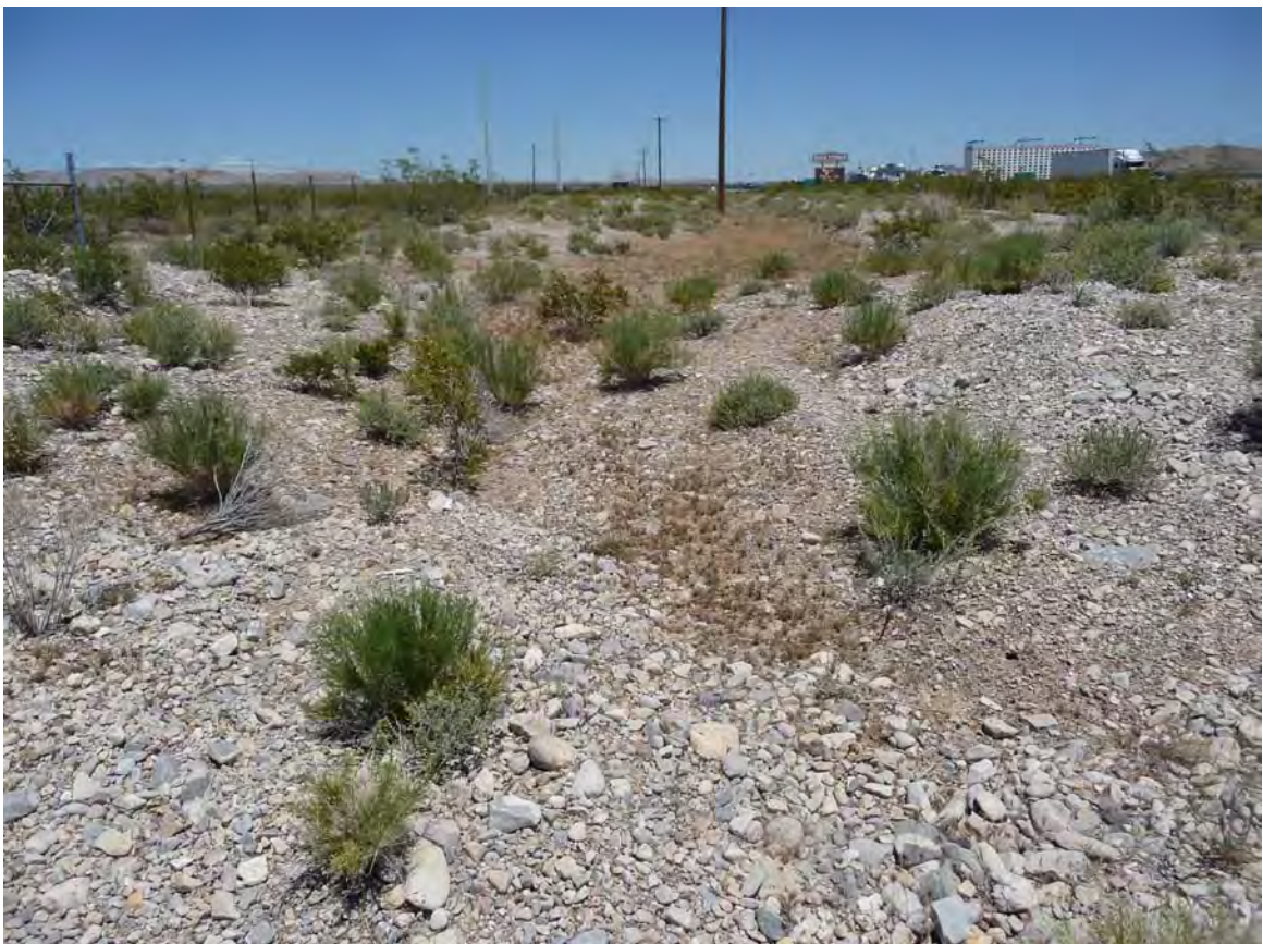
Exhibit A. Figure 30. Manmade drainage connecting to road culvert within HUC 8 Ivanpah-Pahrump Valleys Watersheds / HUC 12 Town of Jean -Frontal Ivanpah Lake Subwatershed
