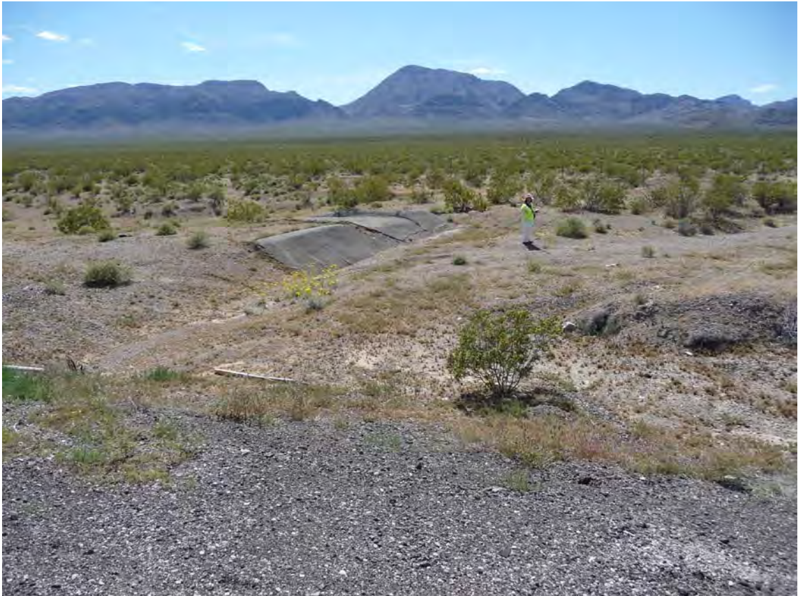
Exhibit A. Figure 25. Manmade drainage connecting to road culvert within HUC 8 Ivanpah-Pahrump Valleys Watersheds / HUC 12 Porter Wash -Frontal Ivanpah Lake Subwatershed
