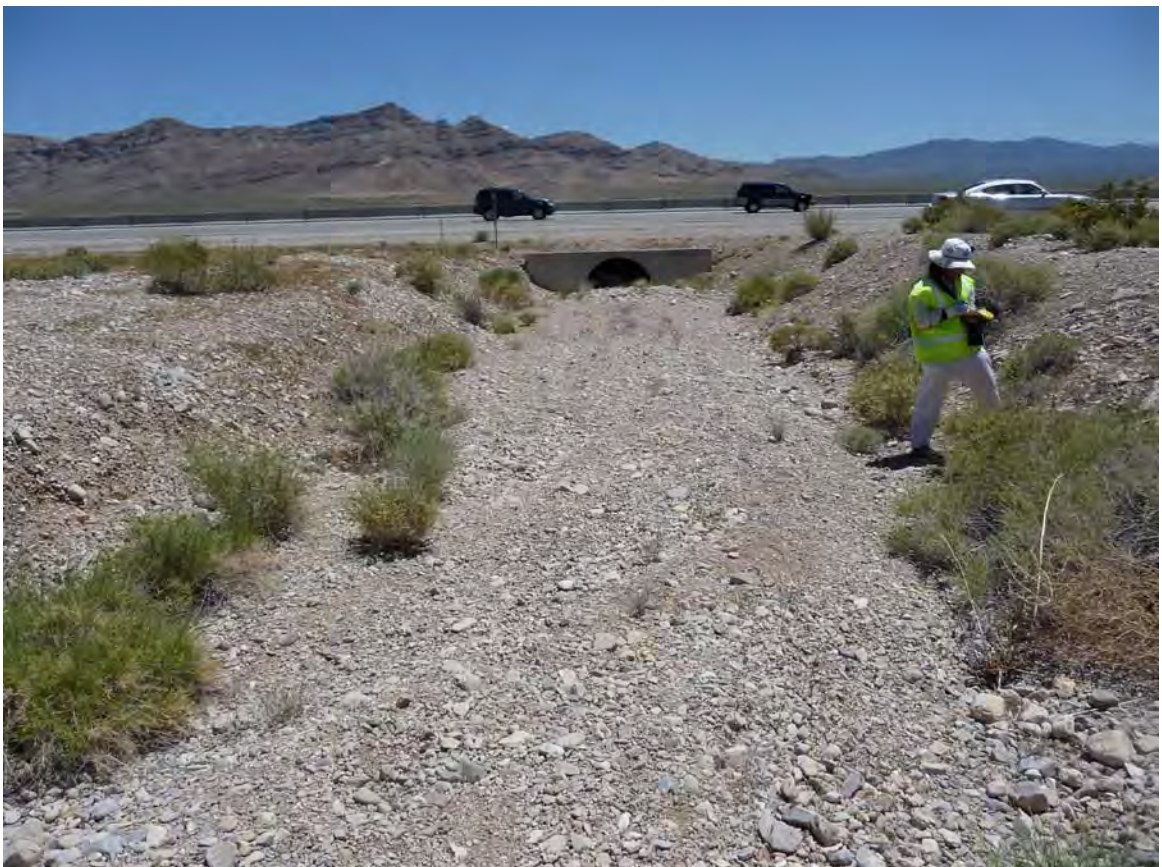
Exhibit A. Figure 34. Manmade drainage connecting to road culvert within HUC 8 Ivanpah-Pahrump Valleys Watersheds / HUC 12 Town of Jean -Frontal Ivanpah Lake Subwatershed
