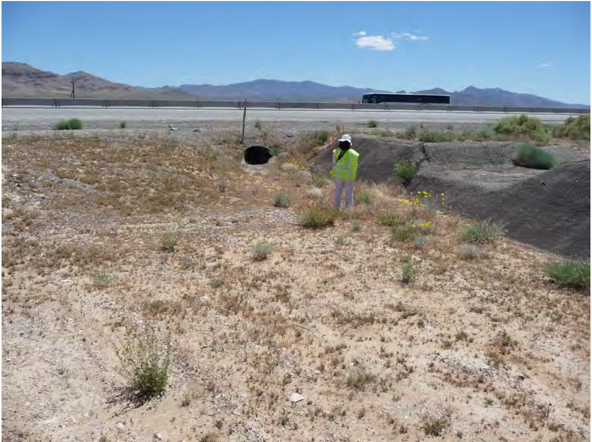
Exhibit A. Figure 31. Manmade drainage connecting to road culvert within HUC 8 Ivanpah-Pahrump Valleys Watersheds / HUC 12 Town of Jean -Frontal Ivanpah Lake Subwatershed
