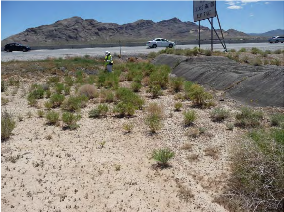
Exhibit A. Figure 29. Manmade drainage connecting to road culvert within HUC 8 Ivanpah-Pahrump Valleys Watersheds / HUC 12 Town of Jean -Frontal Ivanpah Lake Subwatershed
