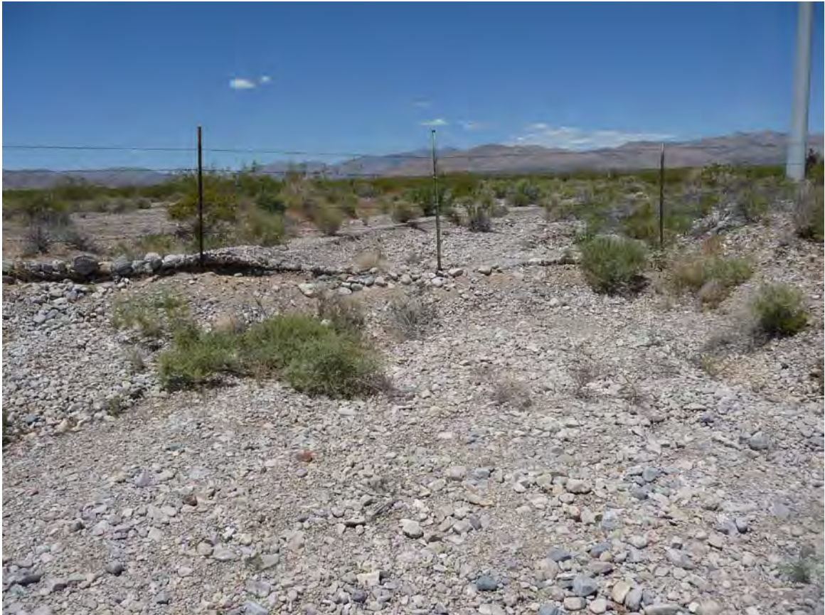
Exhibit A. Figure 33. Manmade drainage connecting to road culvert within HUC 8 Ivanpah-Pahrump Valleys Watersheds / HUC 12 Town of Jean -Frontal Ivanpah Lake Subwatershed
