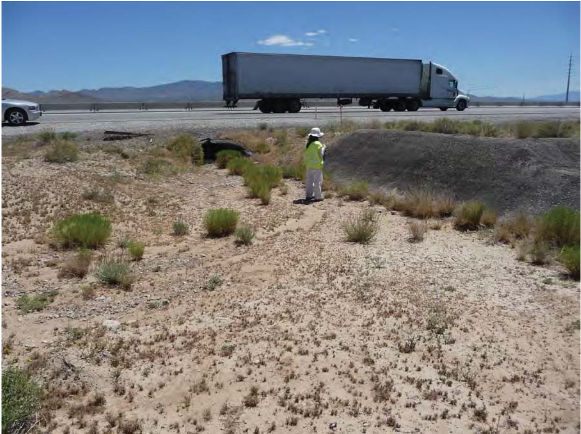
Exhibit A. Figure 35. Manmade drainage connecting to road culvert within HUC 8 Ivanpah-Pahrump Valleys Watersheds / HUC 12 Town of Jean -Frontal Ivanpah Lake Subwatershed
