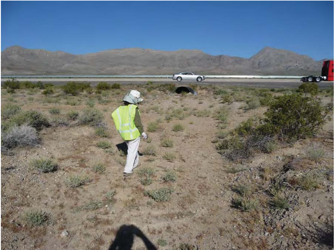
Exhibit A. Figure 23. Ephemeral drainage connecting to road culvert within HUC 8 Ivanpah-Pahrump Valleys Watersheds / HUC 12 Porter Wash -Frontal Ivanpah Lake Subwatershed
