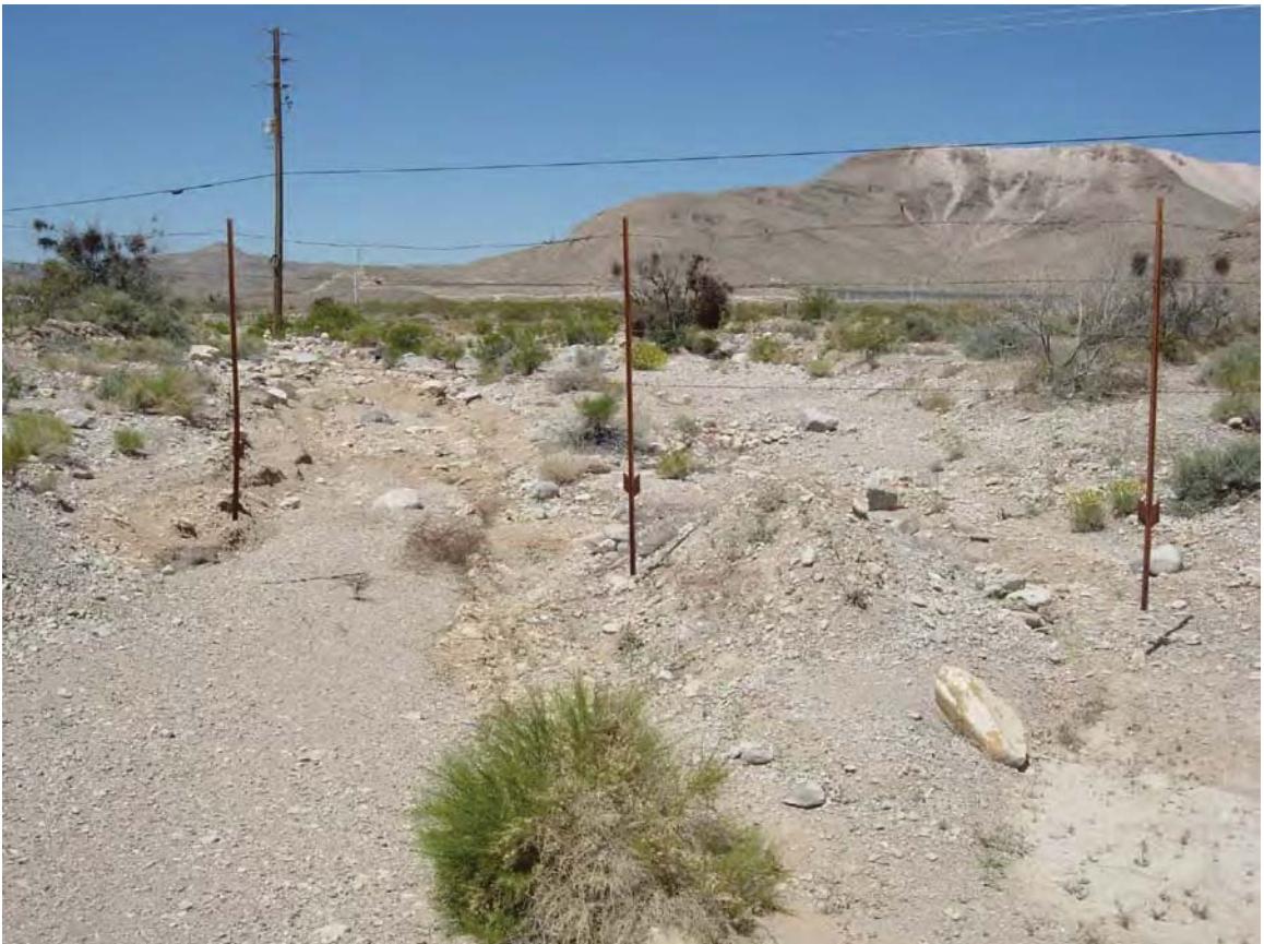
Exhibit A. Figure 23. Manmade drainage connecting to ephemeral drainage within HUC 8 Las Vegas Watershed Wash / HUC 12 Town of Sloan Subwatershed
