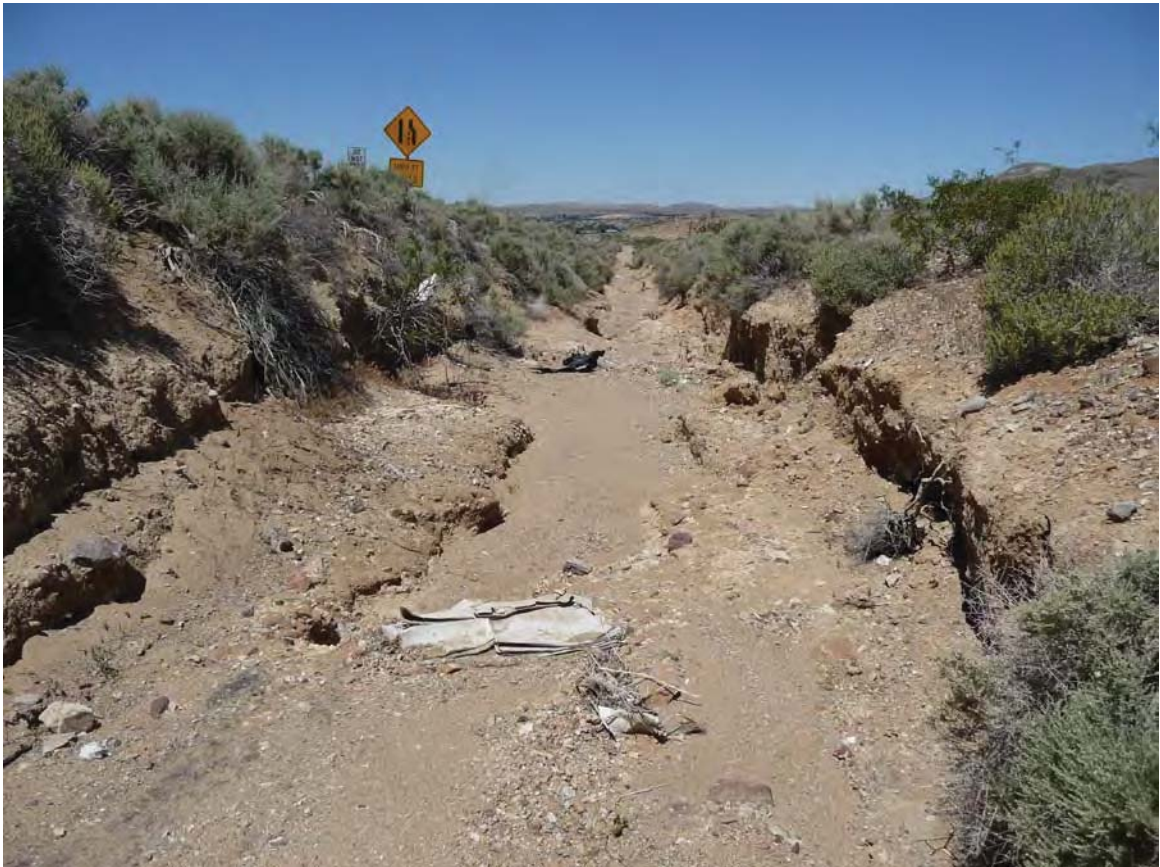
Exhibit A. Figure 21. Manmade drainage connecting to ephemeral drainage within HUC 8 Mojave / Coyote-Cuddeback Lakes Watersheds / HUC 12 City of Barstow - Mojave River Subwatershed
