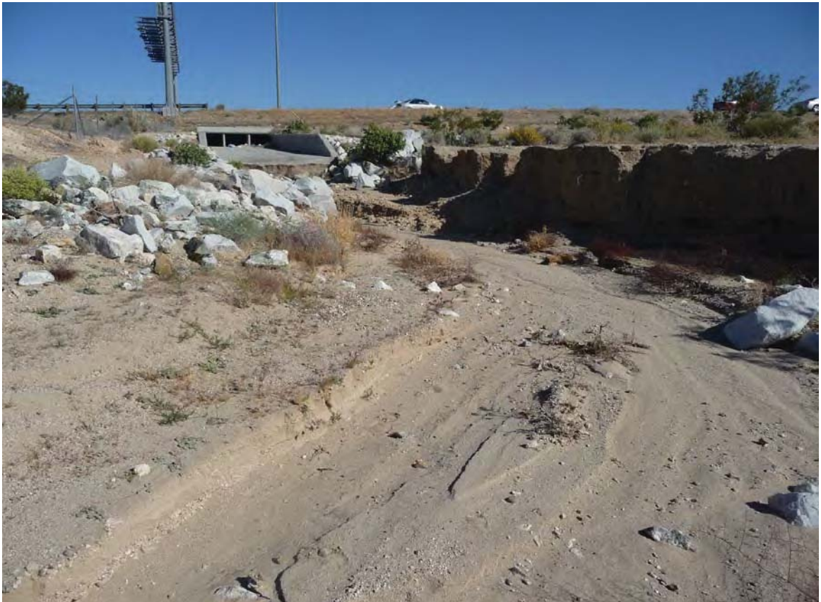
Exhibit A. Figure 18. Manmade drainage connecting to road culvert within HUC 8 Mojave / Coyote-Cuddeback Lakes Watersheds / HUC 12 Town of Lenwood-Mojave River Subwatershed
