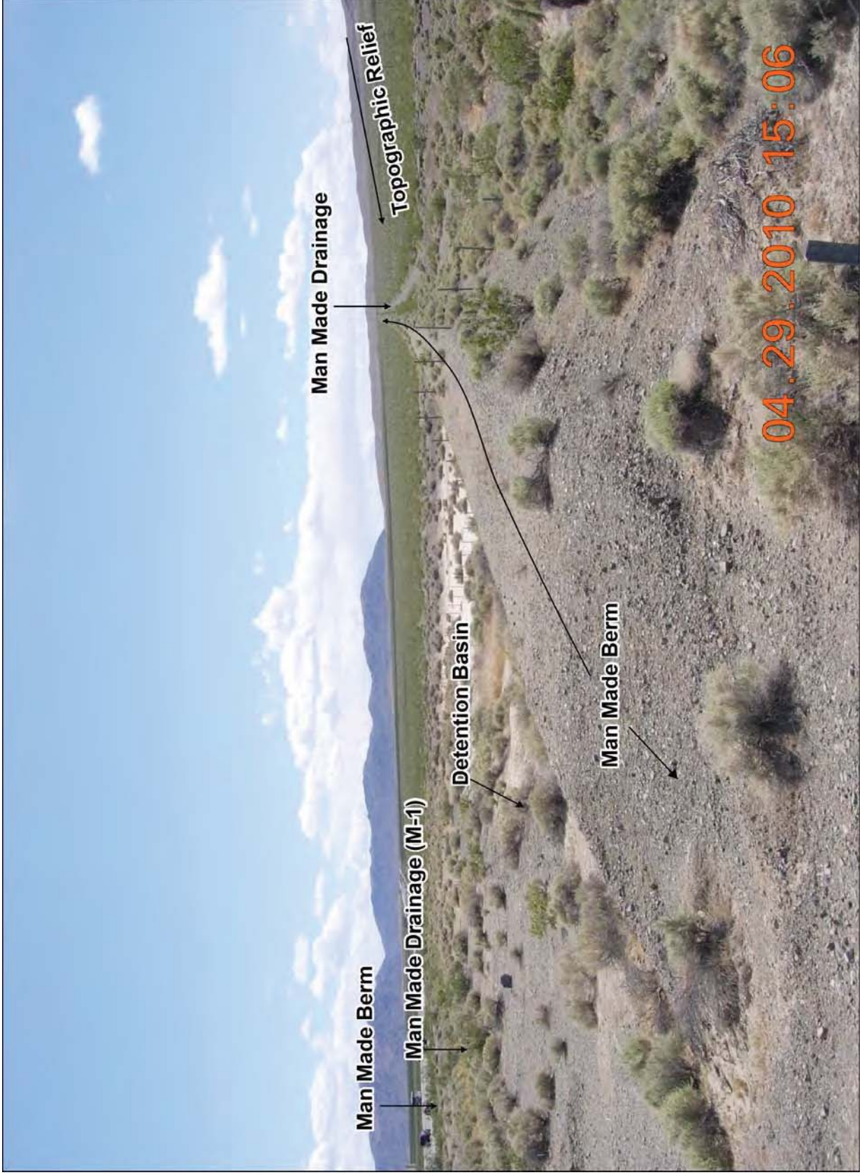
Exhibit A. Figure 10. Typical examples of field indicators of active surface water flow and Ordinary High Water Marks found within ephemerals drainages occurring within the DesertXpress Project Study Area.
