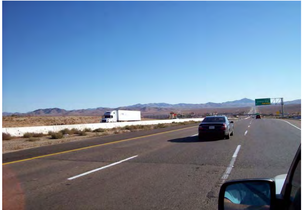
Photograph No. 11: Looking south at southbound I-15 just north of Lenwood, California.
