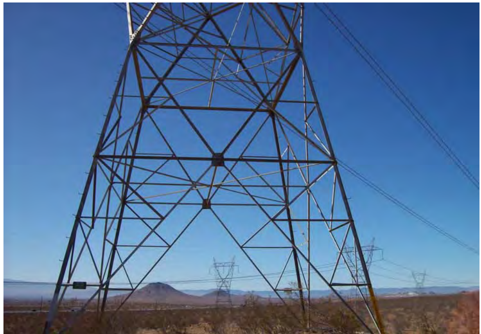
Photograph No. 4: High voltage power lines observed bisecting the site from the north to the south.
