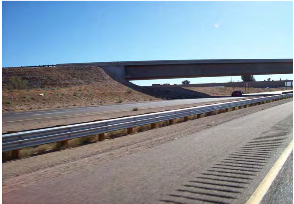
Photograph No. 5: Looking at southbound I-15 median, at Muriel Drive overpass.
