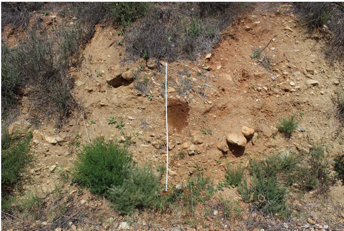
West side road cut along Lytle Creek Road exposing Pleistocene alluvium. Facing southwest.
