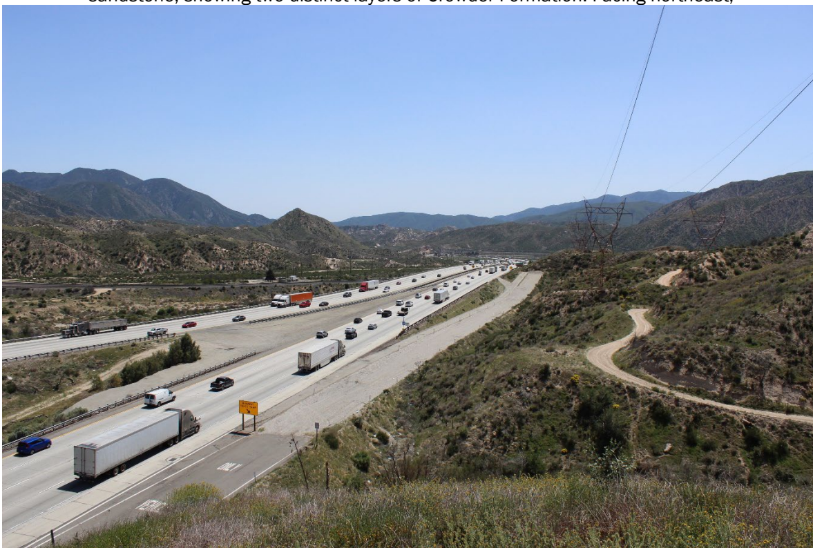
Overview of Interstate 15 through the Cajon Pass. Facing southeast,
