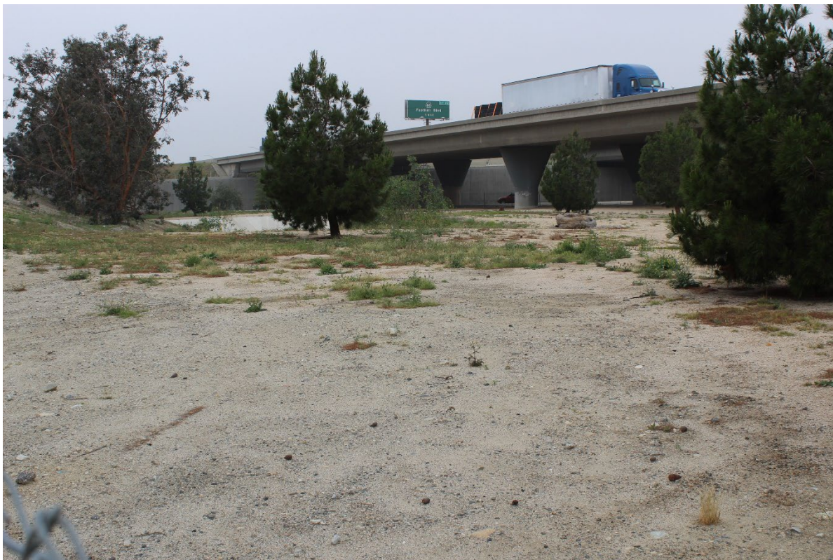
Interstate 15 north off-ramp at Baseline Avenue. Facing southwest
