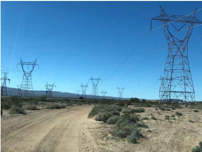
Access road at Segment 1, camera facing southwest toward I-15
