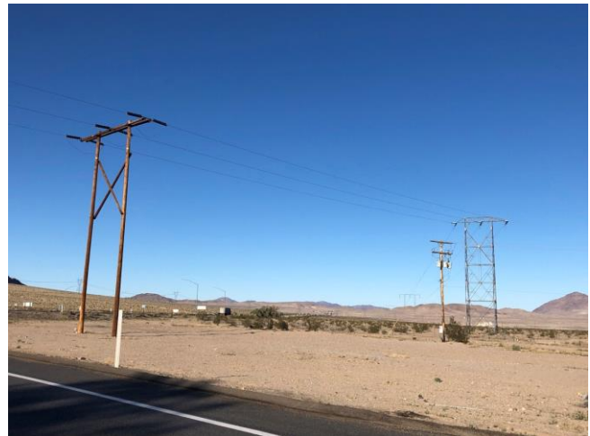
Segment 5, east end, south side. H-frame cross-braced wood pole (foreground, non-contributing), Type A dead-end tower (middle ground, right), Type H tower (background left), camera facing northeast
