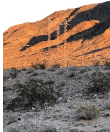
Segment 4, east end, south side. Type AP dead-end tower, camera facing east
