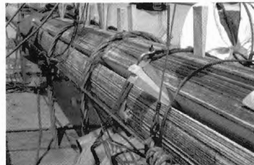
Cable wedged for inspection
