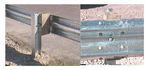
Figure C6-1: Modified G4(1S) guardrail with routed wood blockouts
