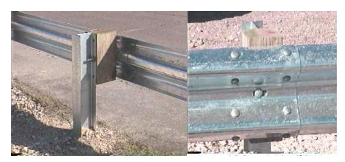
Figure 50. Modified G4(1S) guardrail with routed wood blockouts.
