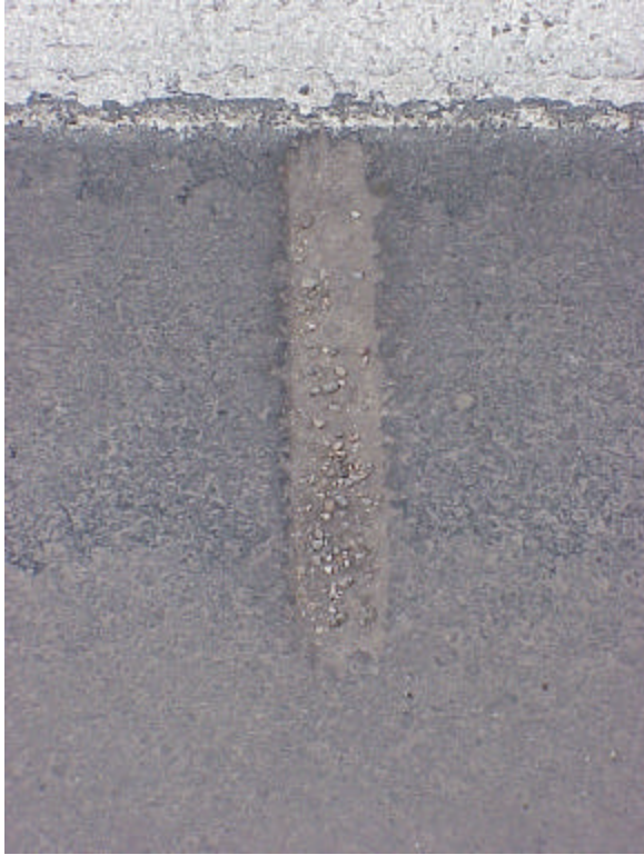
Figure A-3. This two -inch wide groove in section one had trapped a considerable amount of sand and dirt. This photo was taken on March 6, 2001. There had not been any snow on the roadway for several days.
