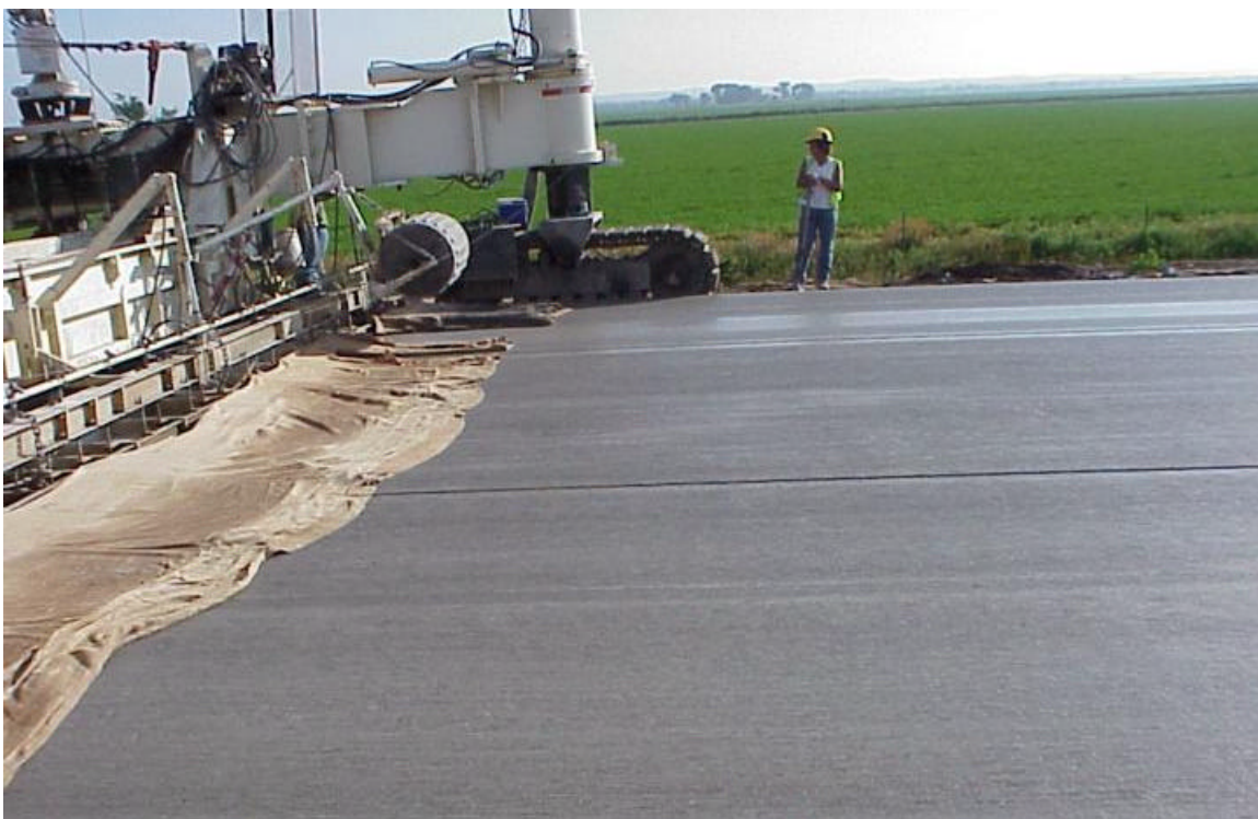
Figure 16. The roller that forms rumble strips in new concrete pavement. The roller that forms the right shoulder rumble strip can be seen at the far side of the paving machine. It has been raised off the surface because the paving operation is approaching an intersection.
