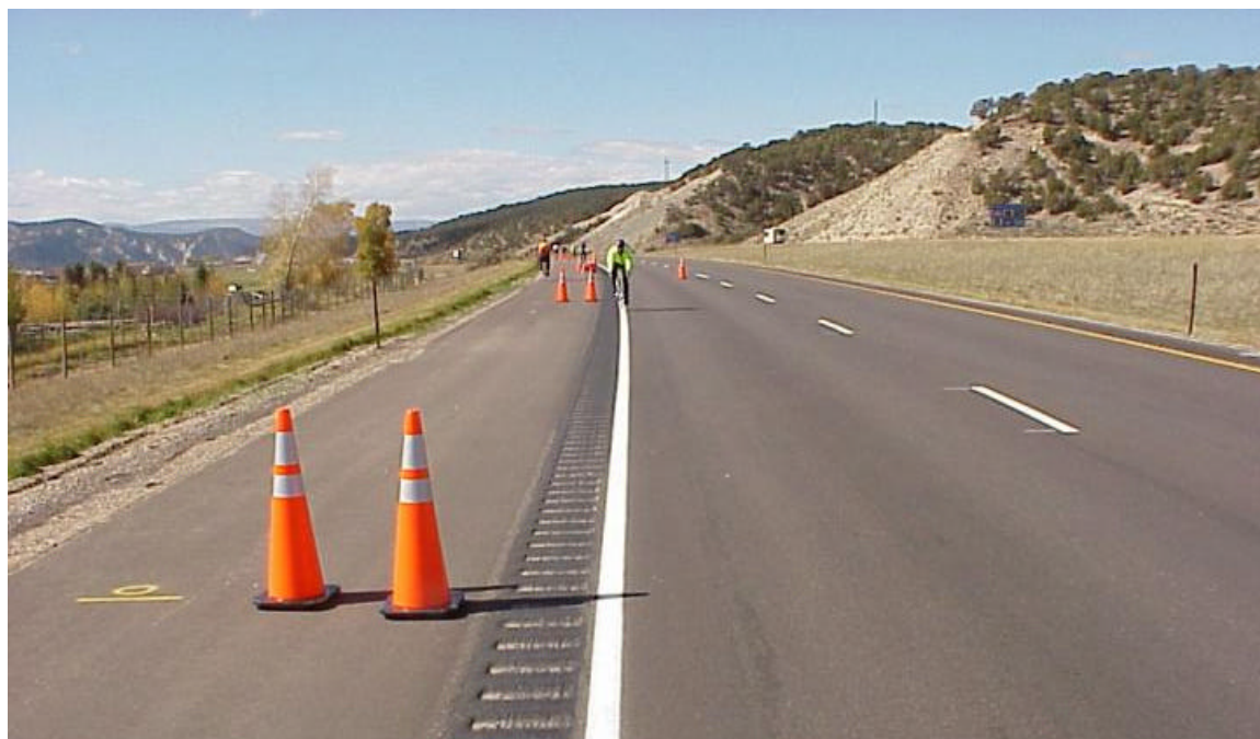
Figure 20. Riders on one of the standard rumble strip sections. The dark stripe over the rumble strip is where CDOT Maintenance crews have applied a sealer to protect the asphalt in the rumble strip grooves. Some of the riders were concerned that this area might become slippery in wet weather.
