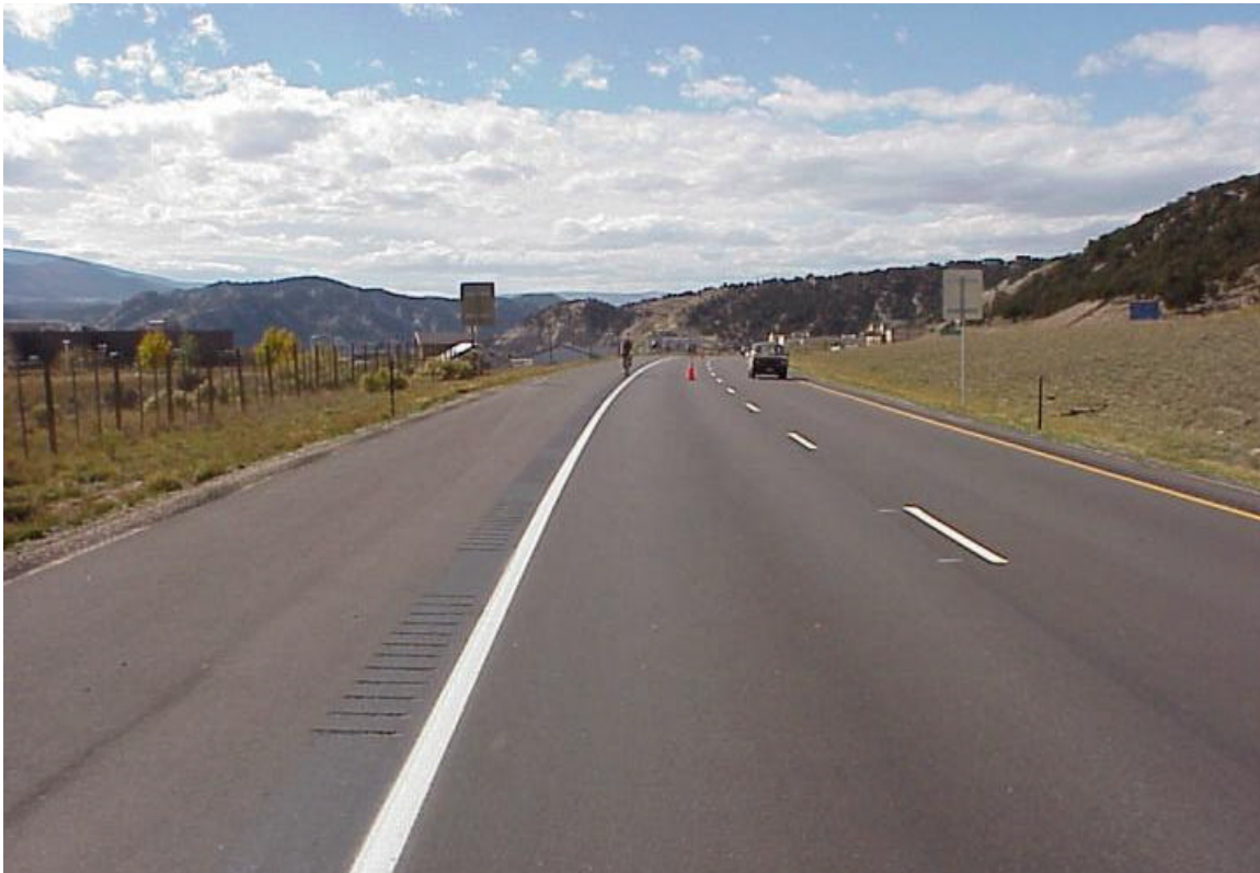
Figure 19. A cyclist on one of the new 2 inch rumble strips. This is a section of interrupted rumble strip
