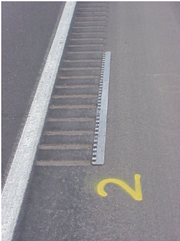
Figure A-6. Section 2 uses 2-inch grooves with 5-inch flats between. This section is continuous rumble strip.
