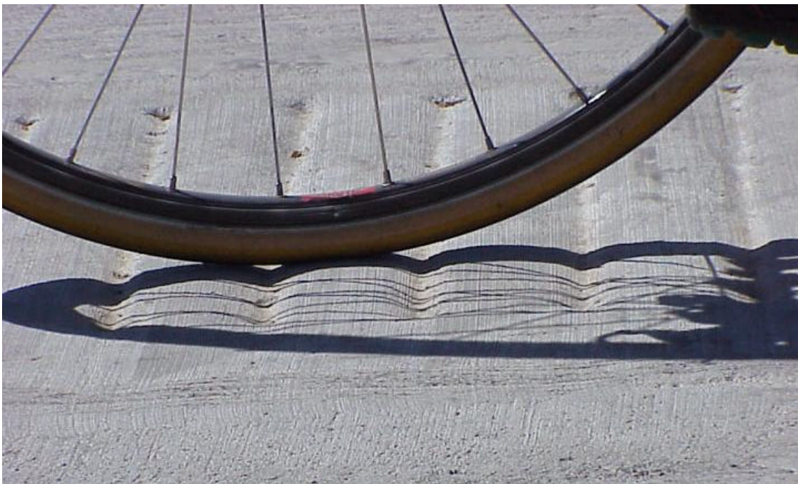
Figure 18. A road bike tire and wheel on a rolled-in concrete rumble strip. The tire has approximately 95 psi air pressure and the riders weight is on the bike. The tire does not sink completely to the bottom of the groove. The rider said this rumble strip would not be a problem for bicyclists.
