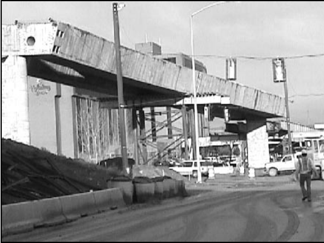
Figure 1.1 I-225/Parker Road Bridge Construction
