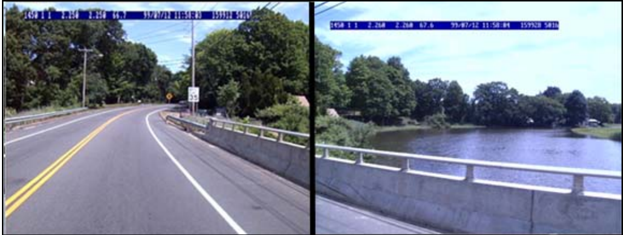
Photo 2. Forward Camera View with Corresponding Side Camera Image
