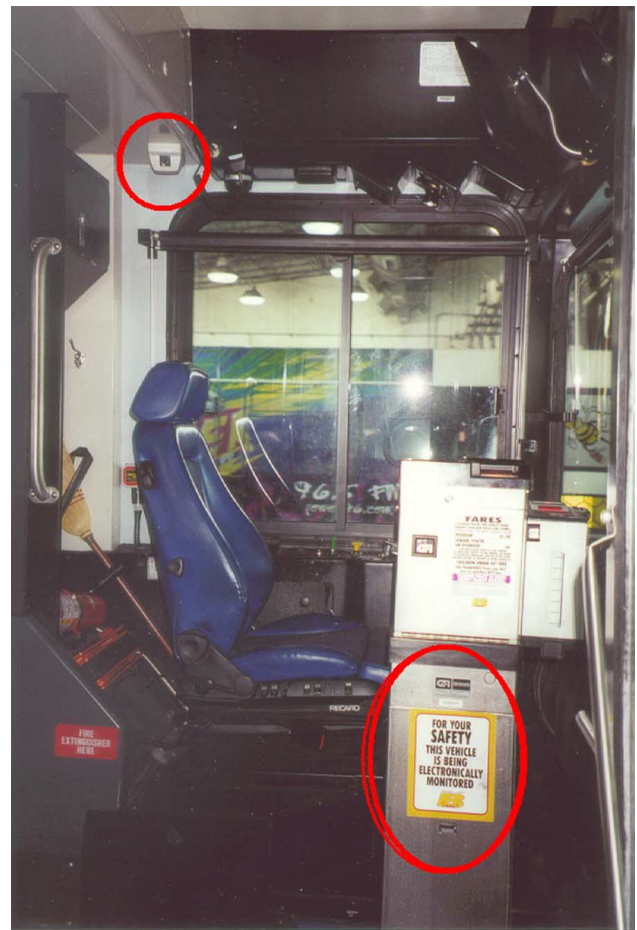
Picture 7 A camera mounted above the operator's seat provides a view of outside activity at a bus stop, boarding customers, and fare payment transactions. Note the sign on the farebox, advising customers they are being monitored.
